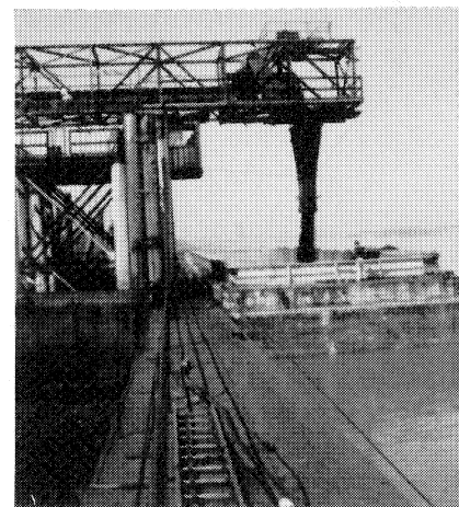
Coal moves from railroad car (not shown) on conveyor belt (top) into barge at American Terminal operated by American Commercial Barge Line Co. on the Ohio River at Louisville, Ky. Coal transfer system is one of four operated by company on Ohio and Mississippi Rivers.
