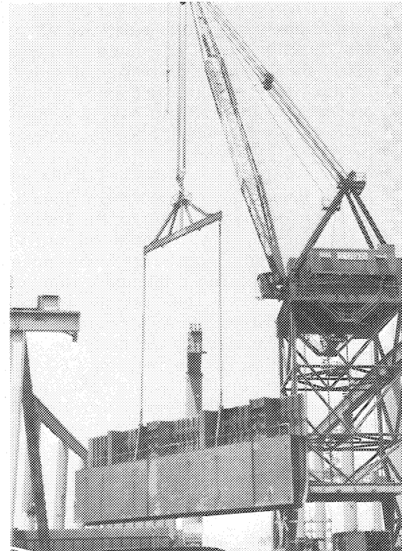
One of the capital improvements at the Los Angeles Division of Todd Shipyards Corp. was the installation of this 175-ton-capacity crane which is used to move large prefabricated sections of a vessel to the building basin.
