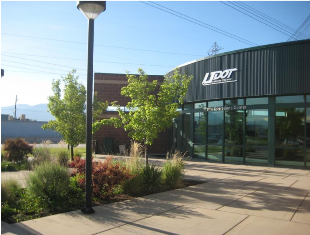
Figure 4.1 Utah DOT Traffic Operations Center
