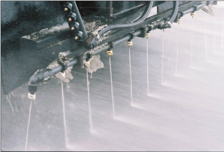
(Photo courtesy of the Oregon Department of Transportation)
