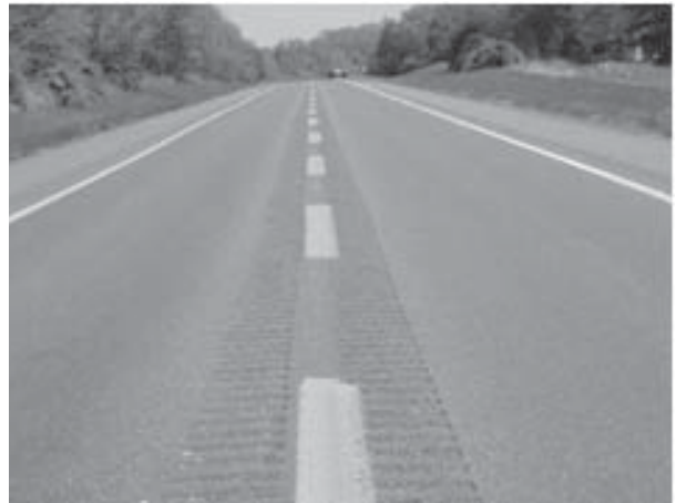
EXHIBIT III-33 Centerline Rumble Strips Implemented in Maryland
