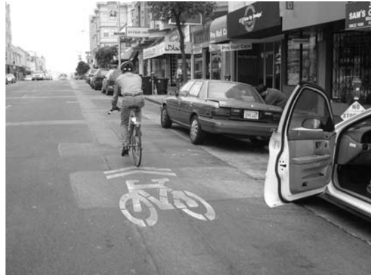
EXHIBIT III-14 Chevron Shared Lane Marking in San Francisco
