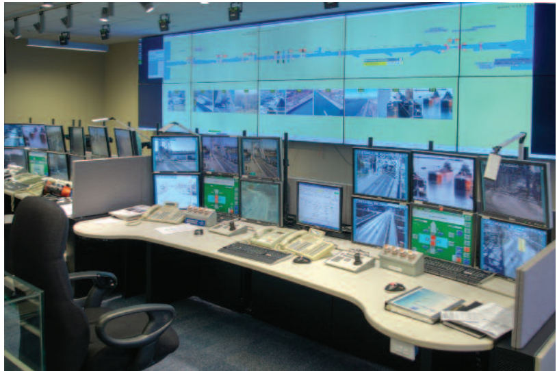
The Niagara Region Operations Control Centre is among a number of traffic control centres that monitor vessels travelling throughout the Great Lakes-Seaway.
