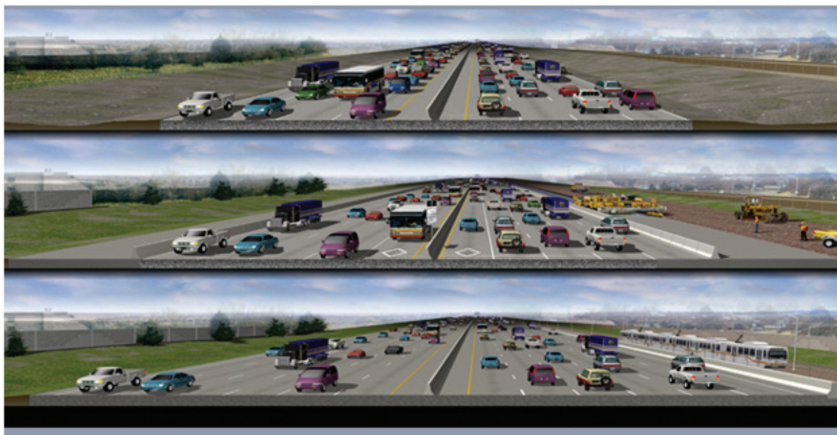
Figure 5.3: HOV Use during I-25 Construction
