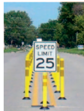
Tubular channelizers in Slater, Iowa
