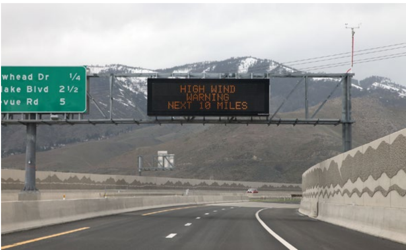
Figure 1. Locations of variable message signs should be selected for maximum effectiveness such as in areas of frequent hazardous weather or traffic incidents and prior to traveler decision points. (Source: Nevada Department of Transportation)
