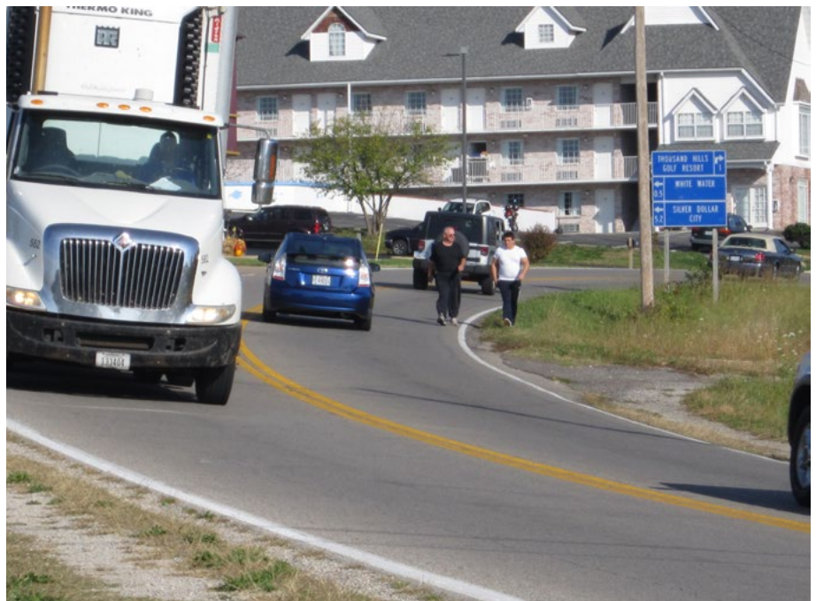
Figure 17. Example of a facility design that did not account for pedestrians or bicycles. (Source: SAIC)
