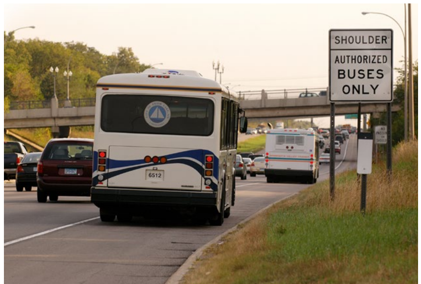
Figure 22. Bus-only shoulder in Minneapolis, MN required site-specific design and operational considerations. (Source: David Gonzales, Minnesota Department of Transportation)
