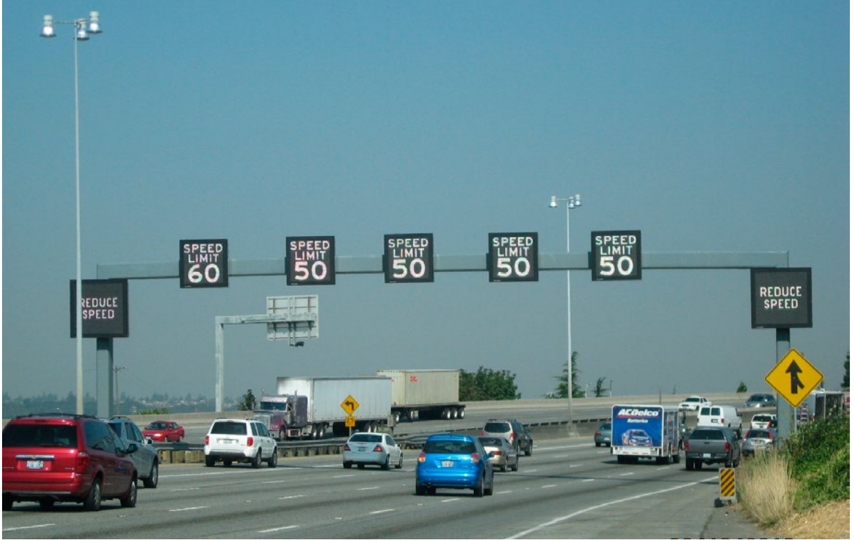
Figure 19. ATM lane control signage on a highway in Washington is placed in a high-visibility location to optimize operations. (Source: Washington State DOT)
