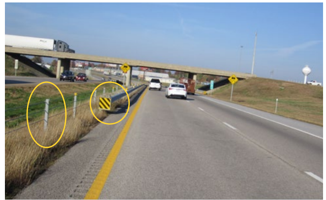
Figure 26. The utilization of two types of median treatments may impact mowing activities. (Source: SAIC)
