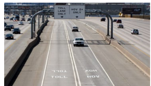
Figure 21. Colorado I-25 HOT lanes enforcement shoulder. (Source: Myron Swisher)
