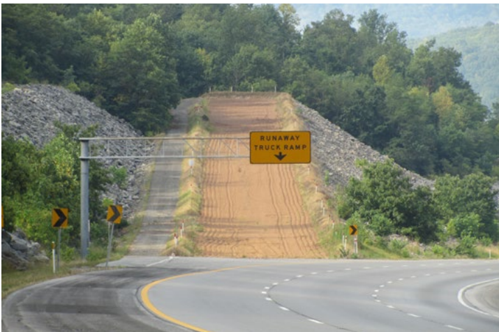
Figure 13. Runaway truck ramp on Interstate 24 in Tennessee, a design element that supports highway operations. (Source: Tennessee Department of Transportation)
