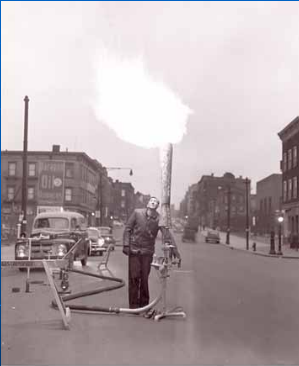
A purge burner igniting manufactured gas being replaced in a main by natural gas during the 'great conversion' in 1952
