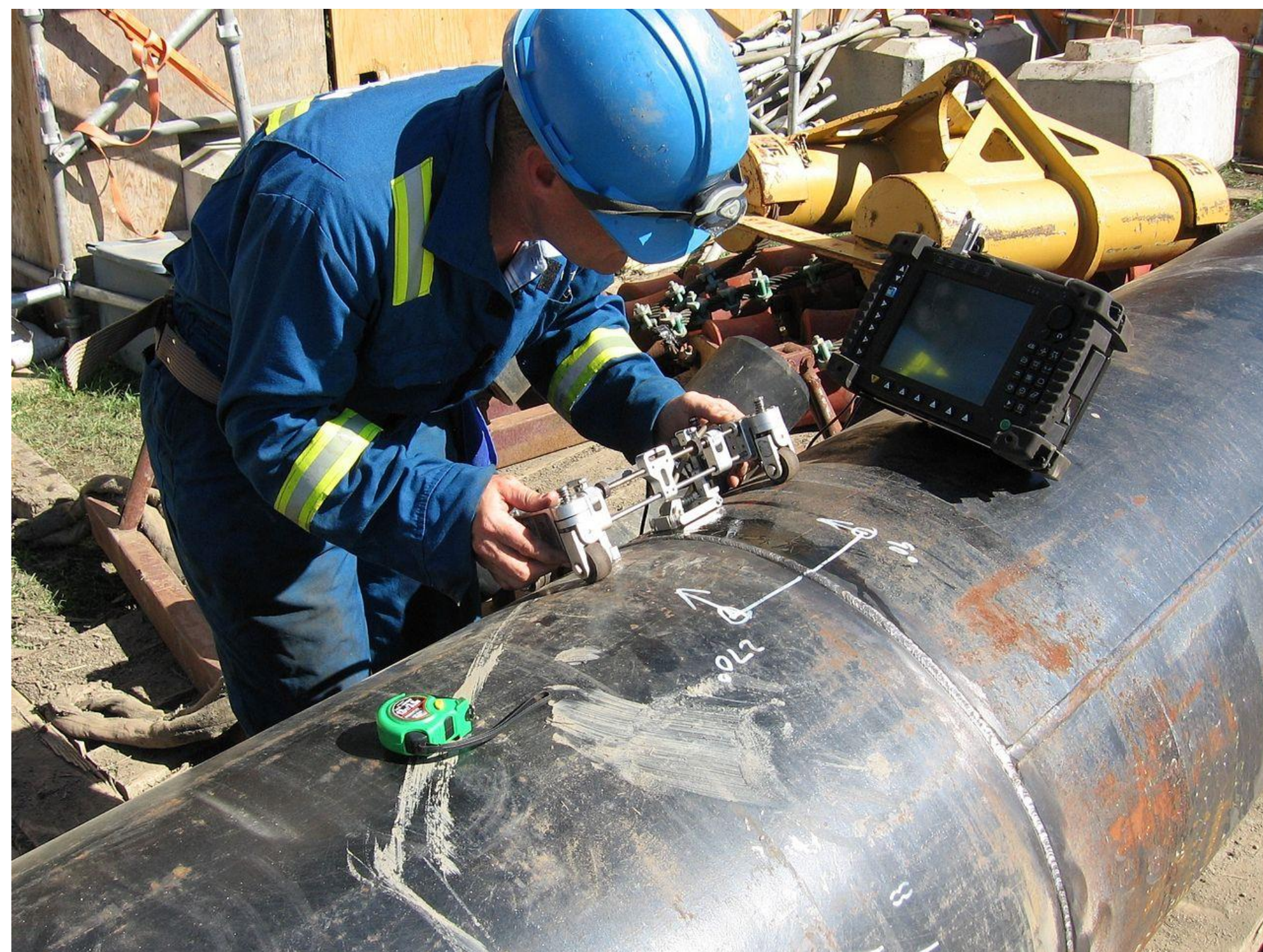
Figure 1. Ultrasonic pipeline inspection.
