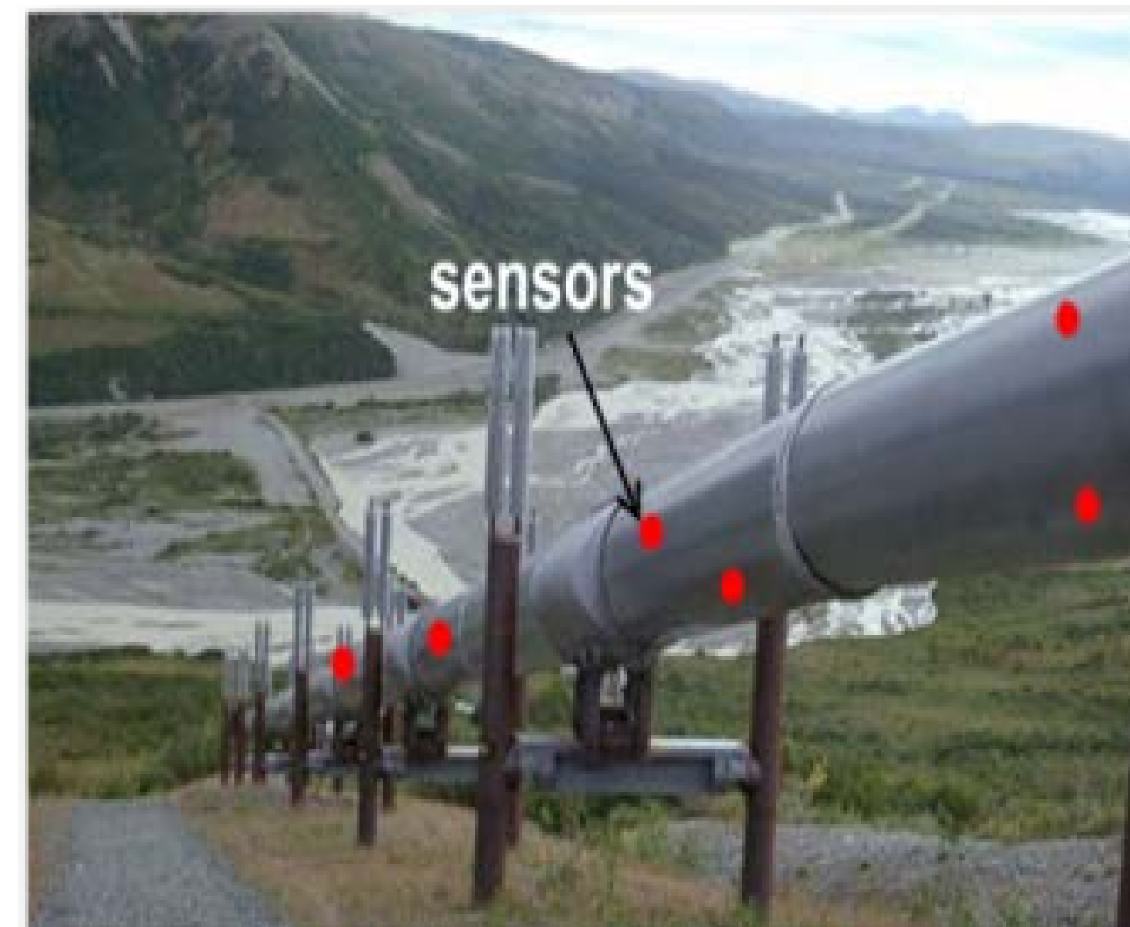
Figure 2. Potential Solution: Structural Health Monitoring (SHM) System
