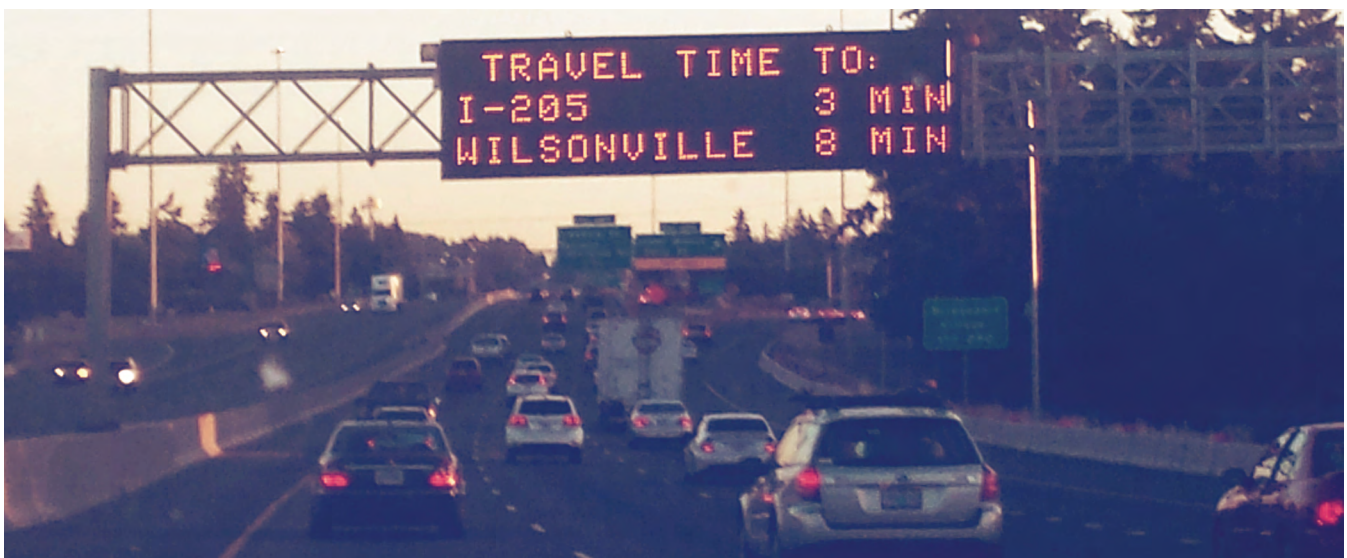
Objectives to improve travel-time reliability may include strategies such as dynamic messaging signs. Photograph courtesy of Kittelson & Associates, Inc.
