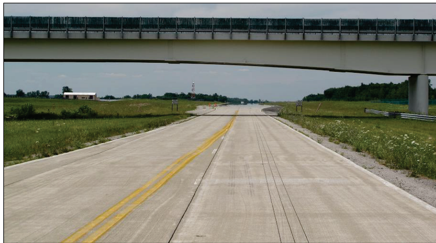
Figure 2.6. A Driver’s View of the Overhead Bridge.
