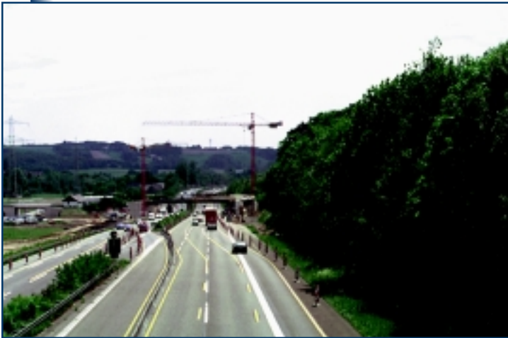
Figure 3. Germany uses yellow markings to delineate travel lanes in work zones; the white markings are left in place, and motorists are taught that yellow markings take precedence over white markings.
