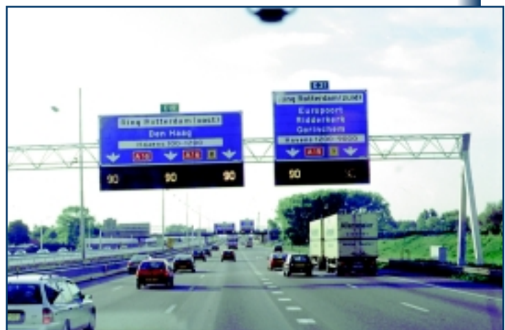
Figure 6. Overhead signs are extensively used in the Netherlands to communicate with motorists. Speed limits change in response to actual travel conditions.
