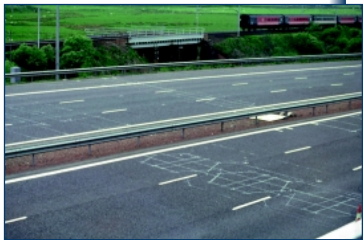
Figure 2. An extensive series of detector loops continually collects information on traffic volumes and speeds on the A6 highway in Scotland.
