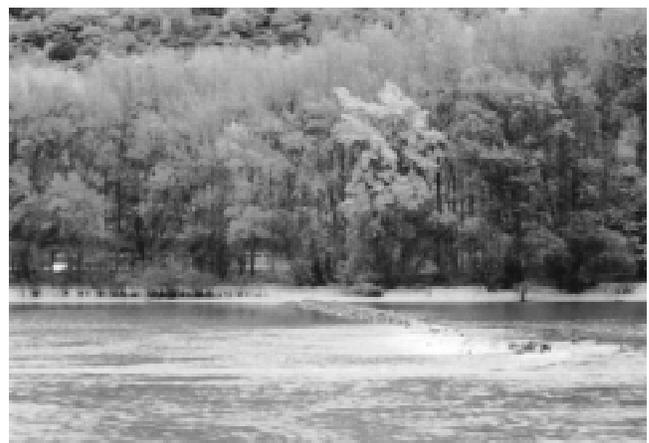
Figure 16. Low rock groin on the Rhine River, Germany.
