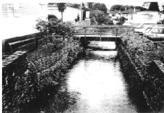
Figure 4. Property close to a river bank limits the choice of strategies for erosion control. Structural solutions, such as gabions, are often the only feasible measure (15).
