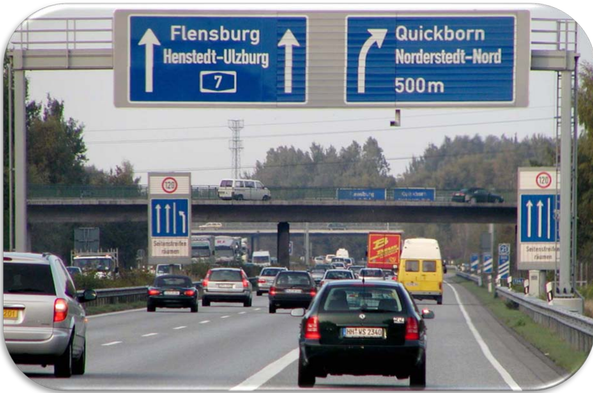
Figure 33. Photo. Termination of Temporary Hard Shoulder Use at Interchange—Germany. (13)
