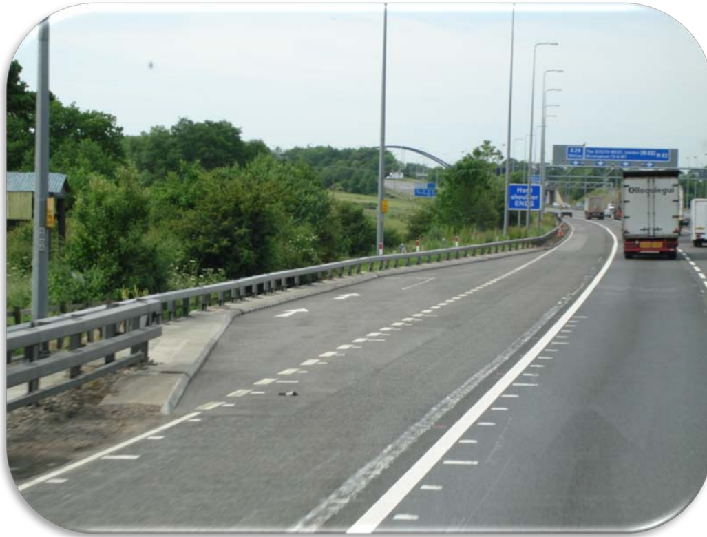
Figure 6. Photo. Shoulder Use with Emergency Refuge Area—Great Britain. (1)
