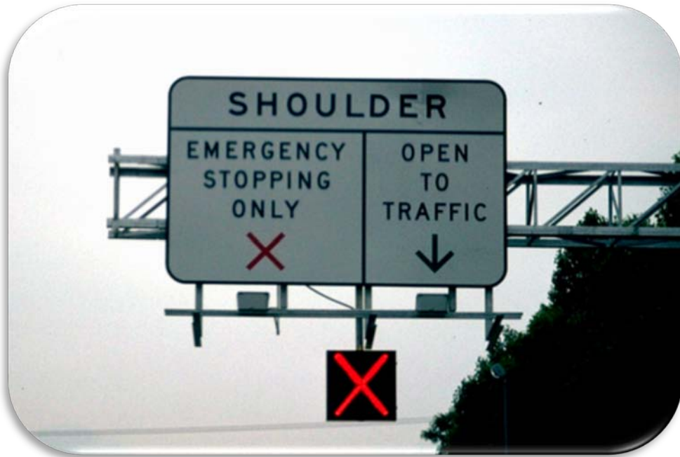
Figure 16. Photo. I-66 Regulatory Sign with Lane Control Signals (Photo Courtesy of VDOT).
