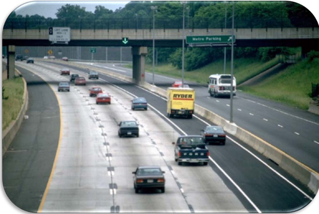
Figure 41. Photo. I-66 HOV/SL Portion—Virginia (50) .
