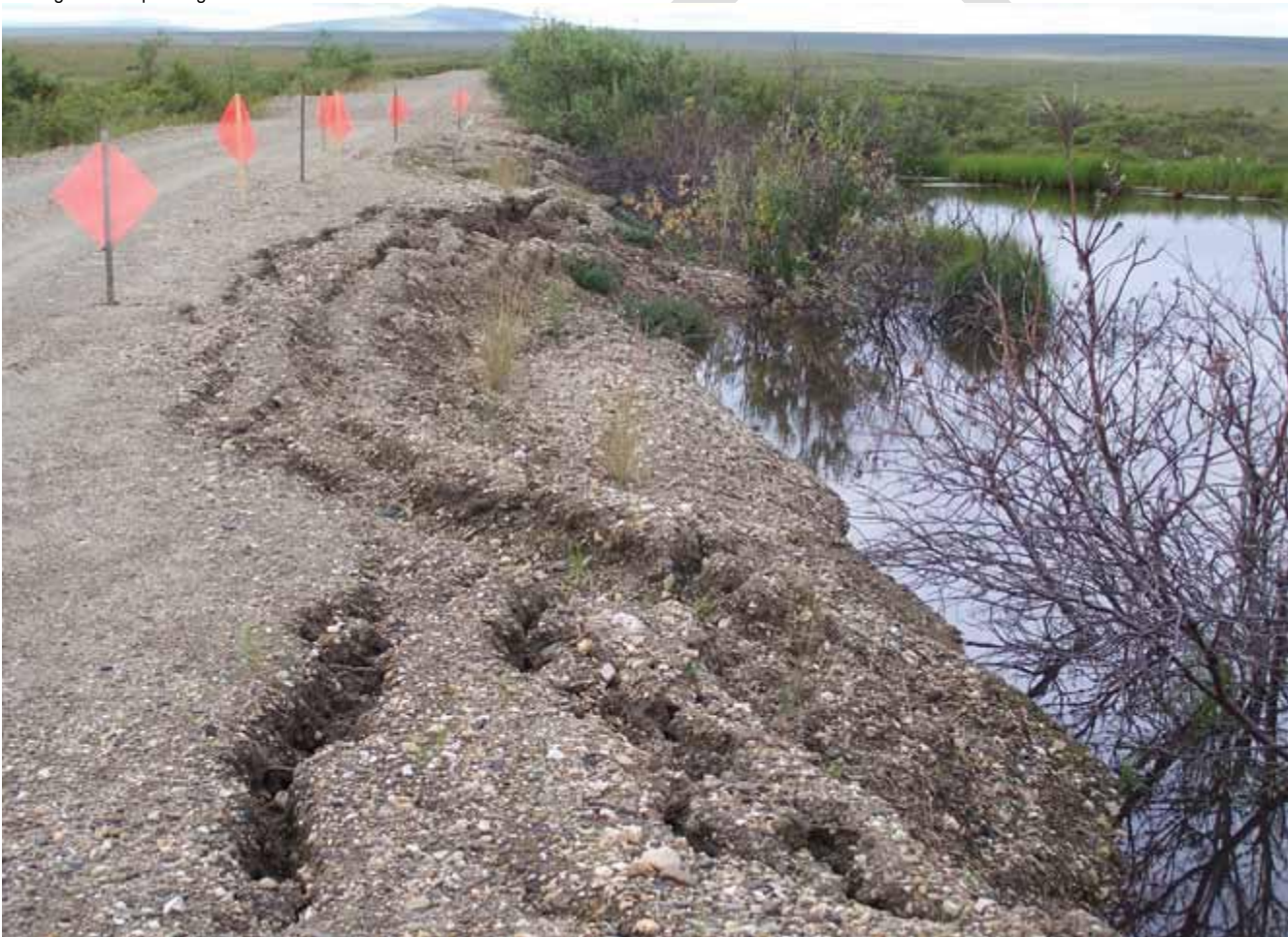
Figure X. Thermokarst formation and road collapse on the Nome to Taylor Highway, outside of Bering Land Bridge (BELA). The pond resulted from thawing and collapse of ground ice.
