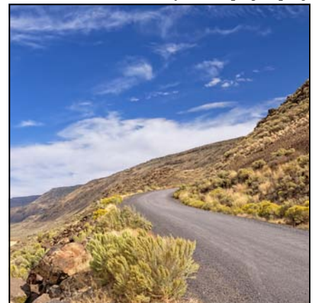
Roadway terraced along hillside at Hart Mountain NWR responds to opportunities and constraints of the topography
