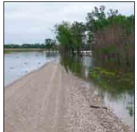
Roads both affect and are affected by hydrology. Floodwaters wash out a road at Flint Hills NWR (top); levee road at Blackwater NWR (bottom).
