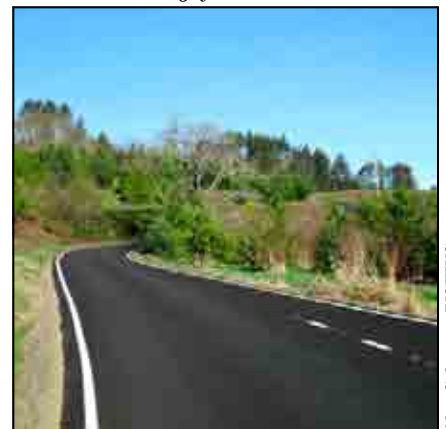
Curving roadway at Nestucca Bay NWR highlights scenery and discourages high speeds (top); emergency personnel respond to an accident at Ridgefield NWR (bottom).
