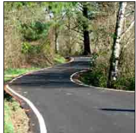
Road alignment at Nestucca Bay NWR preserves upland vegetation and forest.
