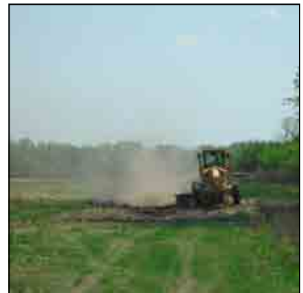
Road construction at Flint Hills NWR.
