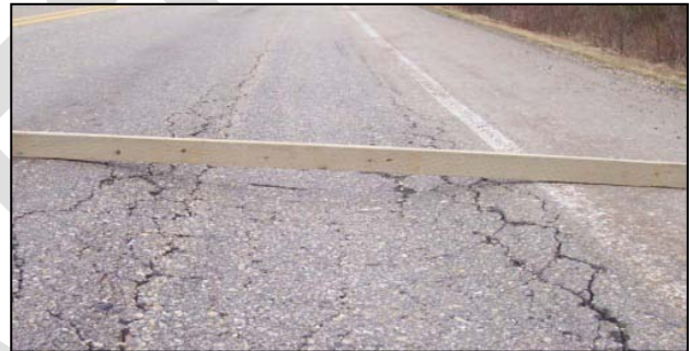
Alaska Highway, damage and rutting (ADOT&PF)
