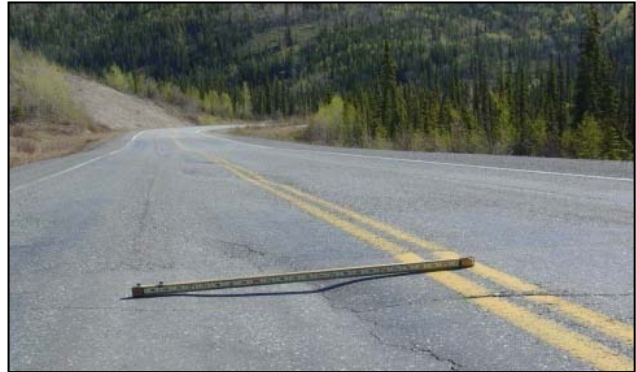
Alaska Highway, damage and rutting (ADOT&PF)
