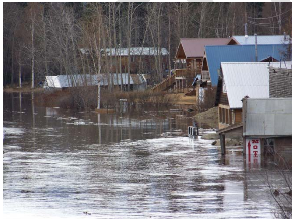
Front Street, flooding (NPS)
