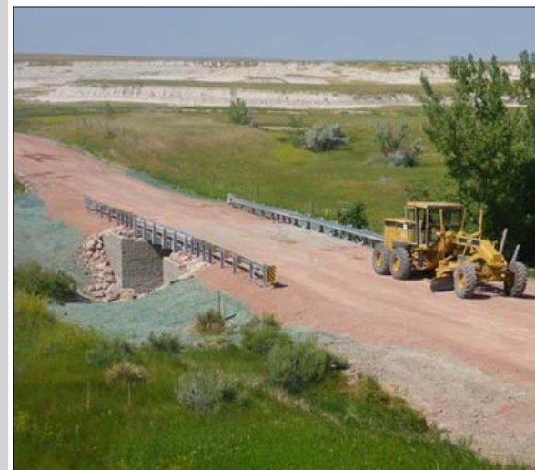
Sand Creek Bridge, During Construction
