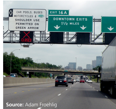
Figure 40. Photo. Use of lane control signals to close lanes on the I-35W PDSL in Minneapolis.
