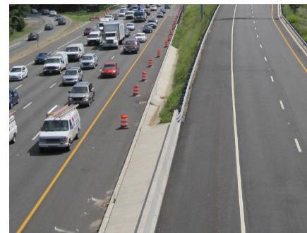
Figure 11. Photo. Permanent physical barrier creates two separate roadways.
