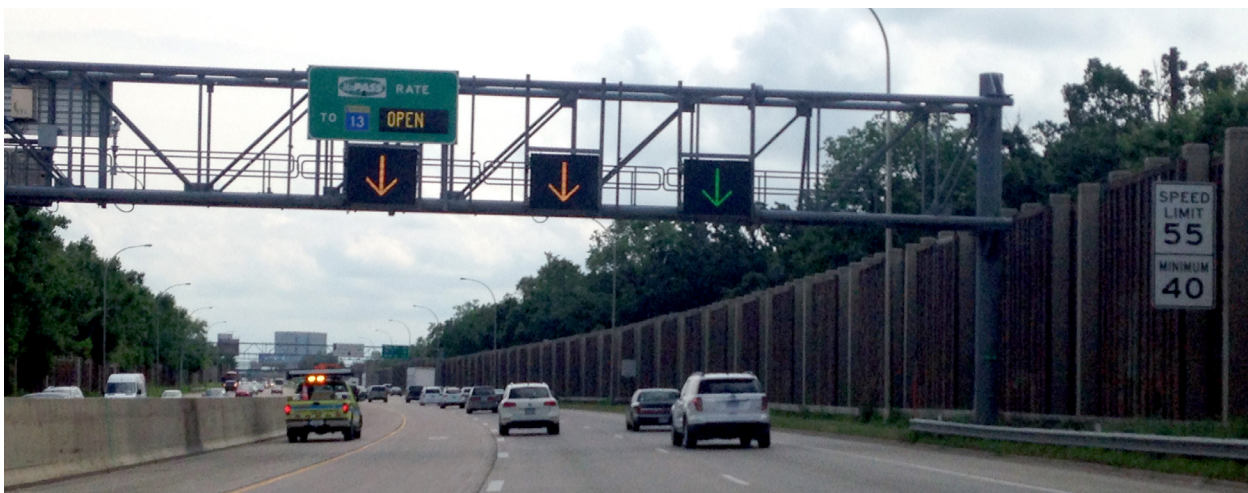
Figure 19. Photo. Managed lanes can suspend all eligibility requirements and allow all traffic.
