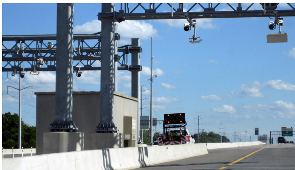
Figure 25. Photo. Enforcement area provides enforcement and service patrol vehicles a safe refuge from traffic.
