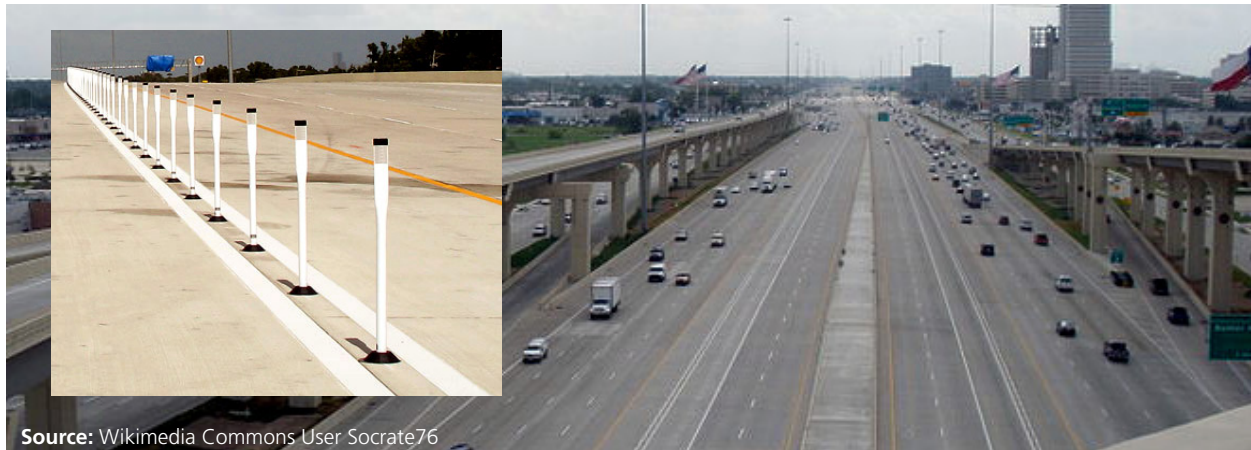
Figure 45. Photo. I-10 Katy Freeway managed lanes with plastic post barrier and full shoulders on either side.
