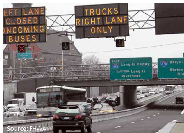
Figure 39. Photo. Effective clearance may be challenging in managed lanes with no shoulders and physical barriers, such as this zipper lane in New York City.
