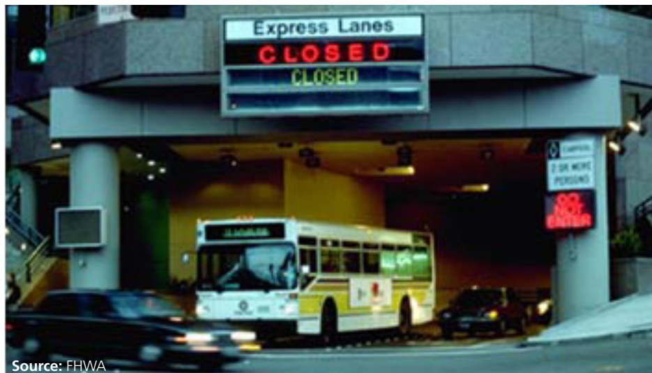
Figure 17. Photo. Some managed lanes can be remotely closed from the TMC, such as this reversible facility.
