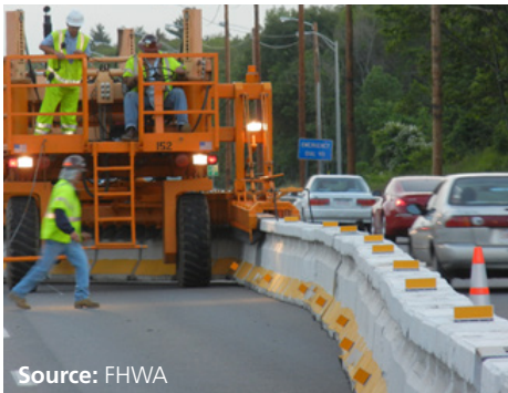
Figure 12. Photo. Zipper barrier and mobile machine.
