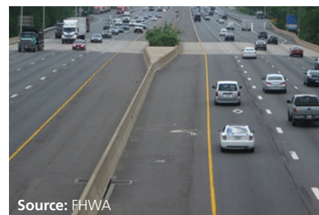
Figure 8. Photo. The left lane is a continuous access HOV lane.
