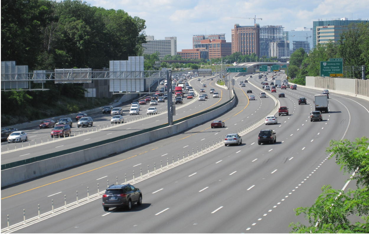
Figure 48. Photo. The I-495 Express Lanes are operated by a private firm and are separated from the publicly owned and heavily congested general purpose lanes by a 4 foot buffer with a plastic post barrier.
