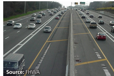
Figure 7. Photo. Managed lane separated from general purpose lanes with painted buffer.
