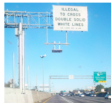
Figure 9. Photo. Invisible electronic barrier using toll tag readers and cameras.
