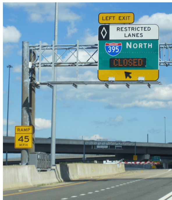
Figure 38. Photo. Some managed lanes have signs and gates that can be used to quickly close the lanes during an incident.
