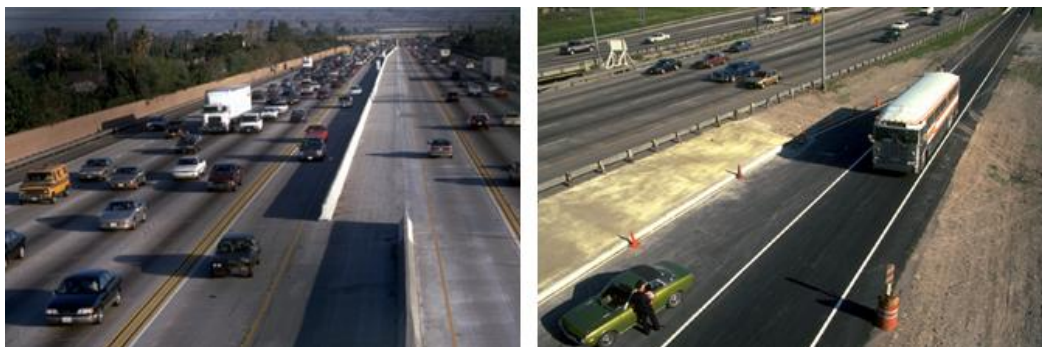
Figure 47: Examples of Enforcement Areas (concurrent flow-left, reversible flow-right)
