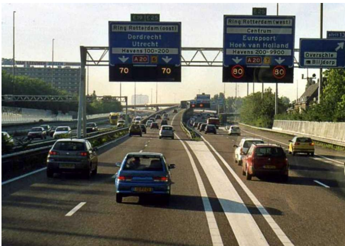
Figure 23: Variable Speed Limit by Lane, Rotterdam, Netherlands
