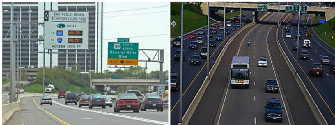
Figure 57: I-394 MnPass Lanes (courtesy Minnesota DOT)
