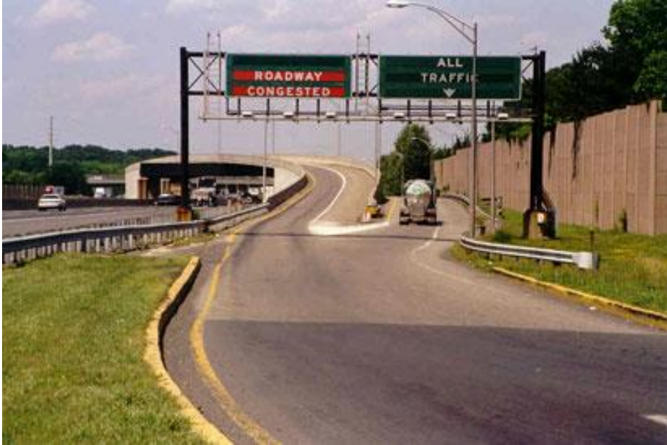
Figure 24: New Jersey Turnpike Queue Warning Signage at Ramp (courtesy New Jersey Turnpike Authority)
