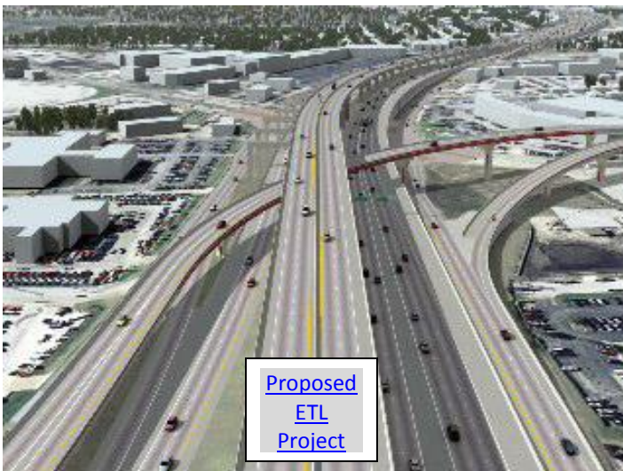
Figure 21: Express Toll Lanes on SH 183/I-820, Ft Worth, Texas (courtesy of North Tarrant Express)
