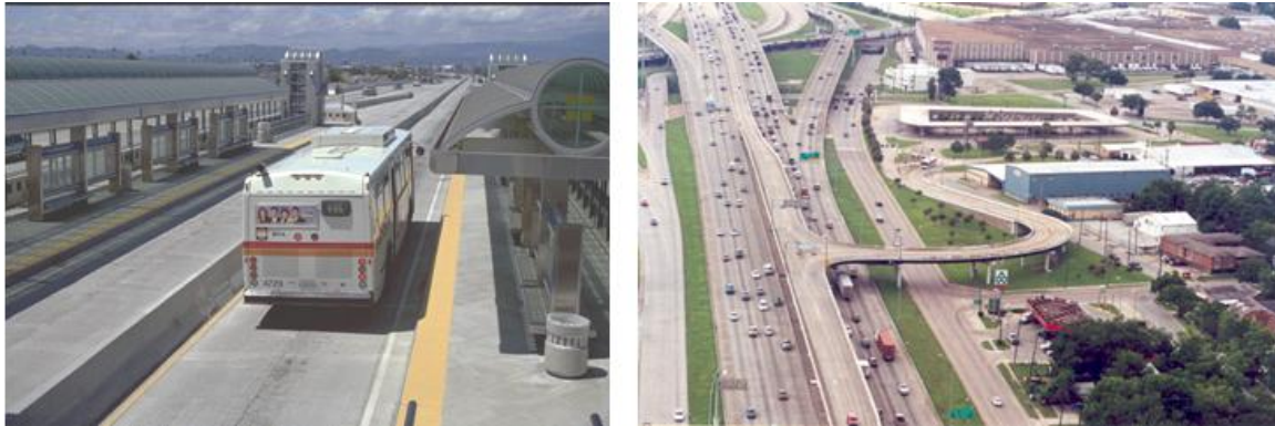
Figure 48: On-Line and Off-Line Transit Stations (I-110 Los Angeles left, I-45 Houston right) (right photo courtesy of Texas Transportation Institute)
