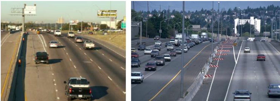
Figure 42: Slip Ramps Providing Terminal Access to Managed Lanes, Dallas, Texas (left) and Seattle, Washington (right) (3)
