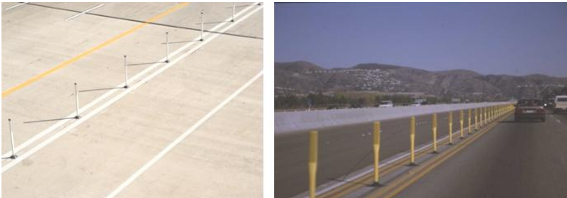
Figure 39: Examples of Pylons Placed in a Wide Buffer (left) and Narrow Buffer (right)
