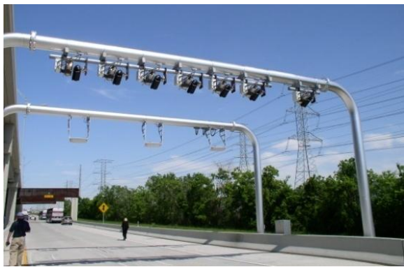
Figure 45: Electronic Toll Collection Gantry with LPR and Sample Transponder.
