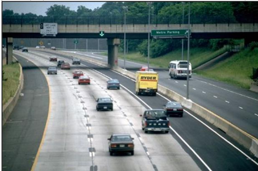
Figure 59: Dynamic HOV Lane (leftmost lane) and Dynamic Shoulder Lane (rightmost lane) on I-66
