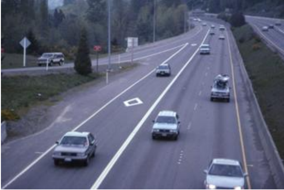
Figure 35: Right Side HOV Lane on I-405, Bellevue, Washington (since reconfigured on left).
