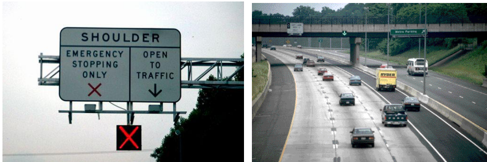
Figure 26: Lane Control Signal on I-66, Virginia Signage over right shoulder lane (left) with leftmost lane restricted to HOVs (right)
