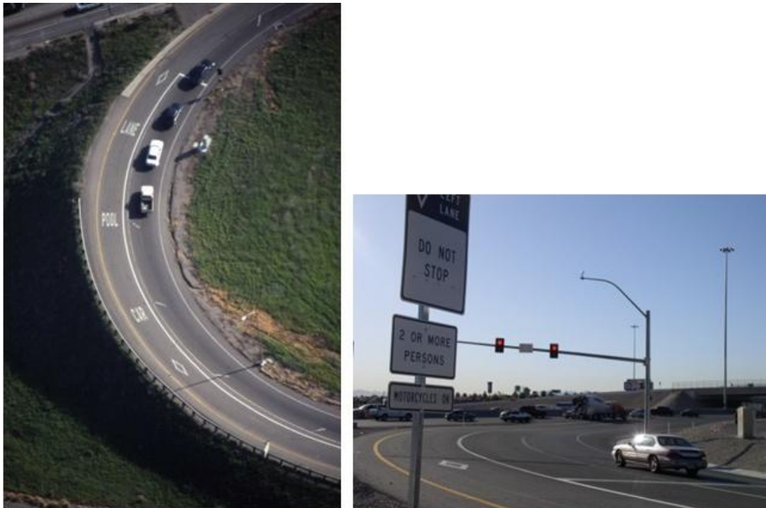
Figure 17: Examples of HOV Ramp Meter Bypasses on Freeways
