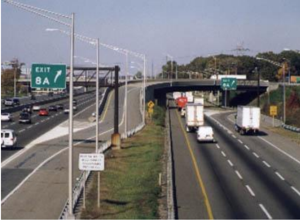
Figure 12: New Jersey Turnpike Dual Roadways Segregating Truck Movements (courtesy New Jersey Turnpike Authority)
