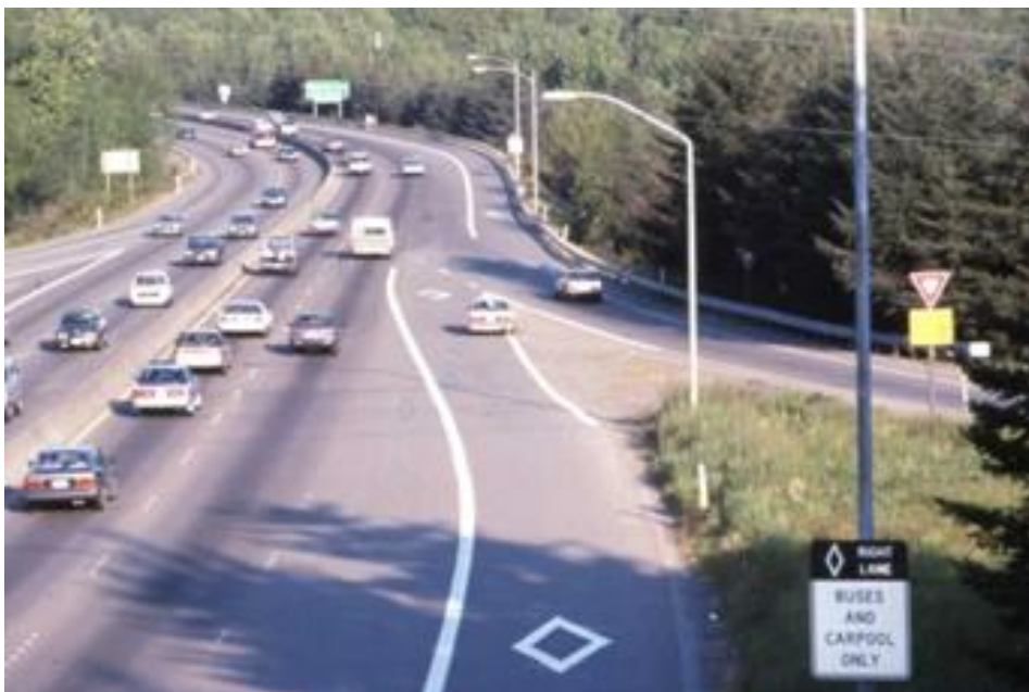
Figure 34: Right Side HOV Lane on SR-520, Bellevue, Washington
