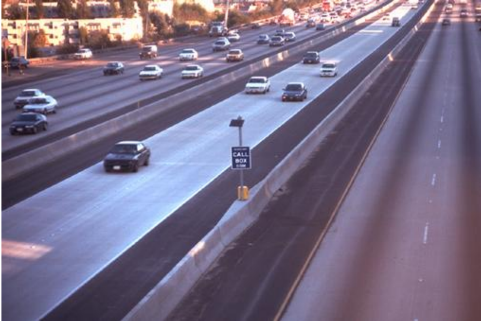
Figure 19: I-15 Express Lanes, San Diego, California
