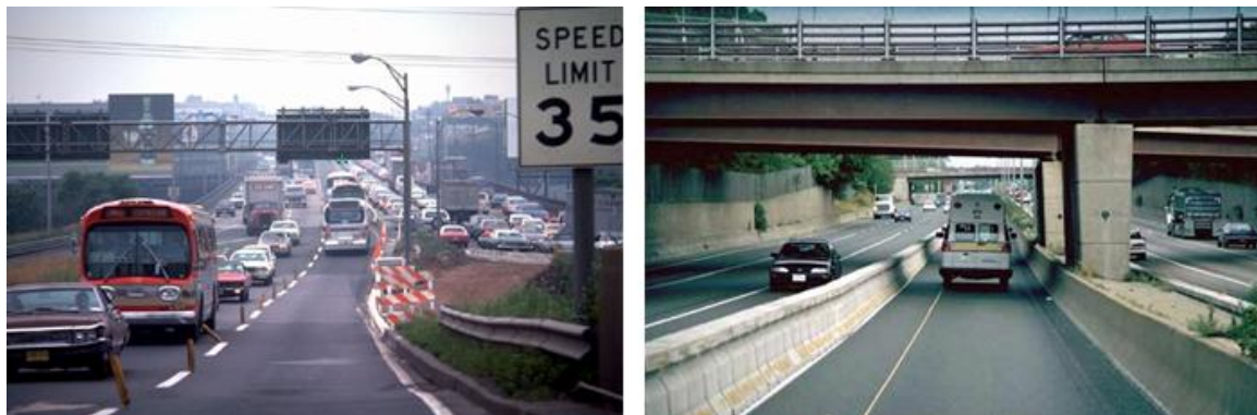
Figure 37: Examples of Contraflow Lanes on Route 495, New Jersey and I-93, Boston, Massachusetts
