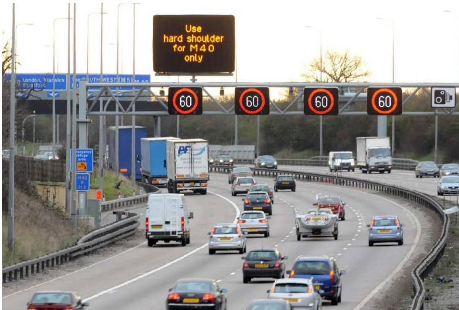
Figure 61: Variable Speed Limit and Dynamic Message Sign, M42 Motorway, Manchester, United Kingdom (courtesy Highways Agency, UK)
