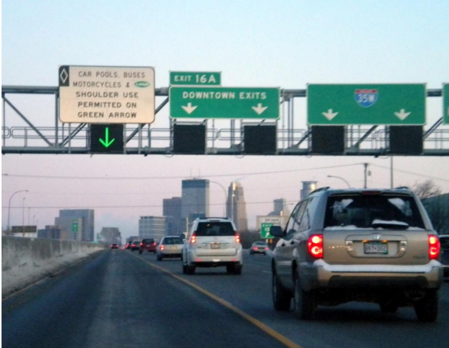
Figure 25: Lane Control Signal over I-35W PDSL, Minneapolis, Minnesota
