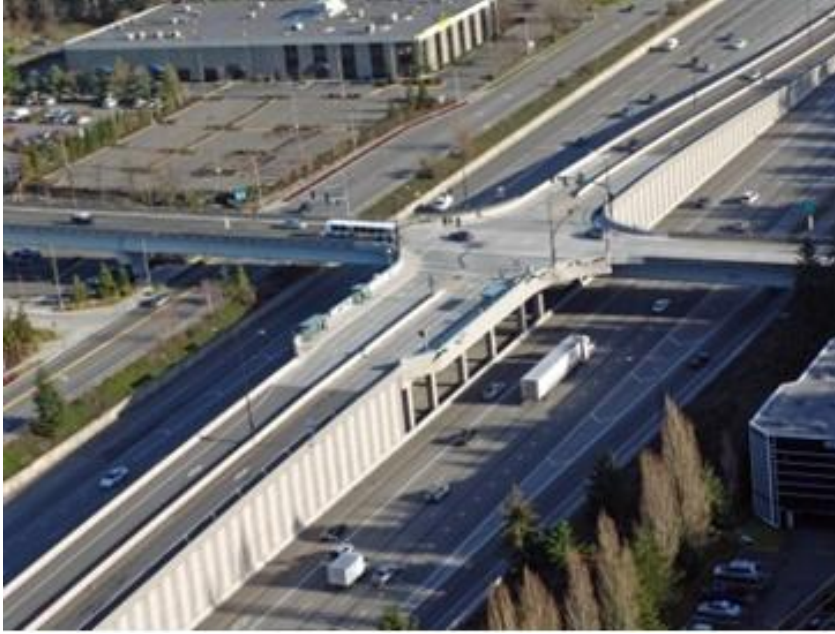
Figure 13: Direct Access Ramp to Concurrent HOV Lanes, Seattle, Washington (courtesy Sound Transit)
