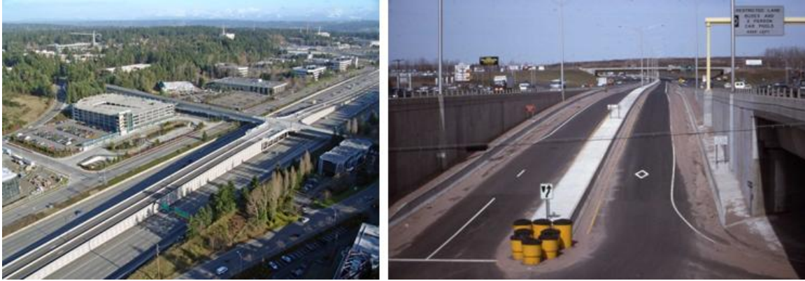
Figure 43: Median Drop Ramps (elevated-left, depressed-right) (left photo courtesy Sound Transit)
