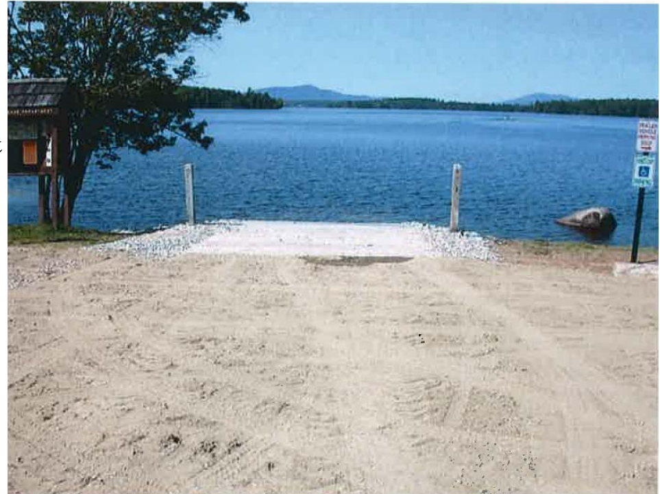
Existing Access condition
