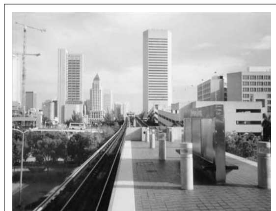
Photo 13.3. View of Government Center Metrorail/Metromover Station from the Overtown Metrorail Station.
