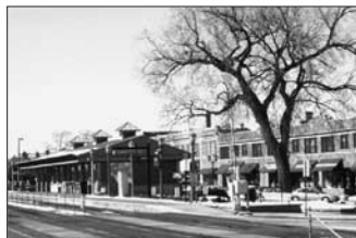
Rehabilitated Metra Station
