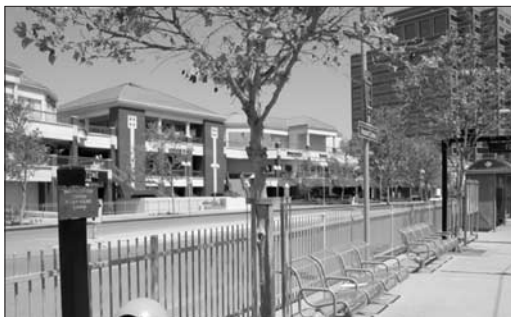
Photo 19.3. Hazard Center’s Shopping Center and 300,000-Square-Foot Office Building. (Northeast of the Hazard Center Station)
