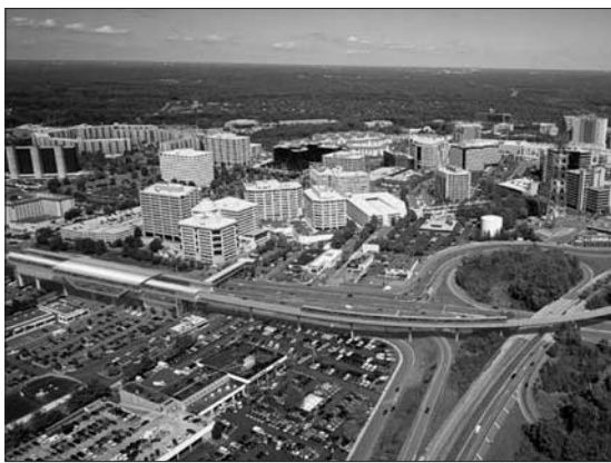
Photo 12.2. Proposed Rail Station Site at Tyson's Corner. Source: Dulles Corner Rapid Transit Project.
