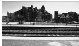
View from the Metra Station
