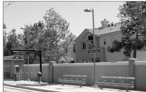
Photo 19.4. Hazard Center’s 120 Condominiums. (South side of the Hazard Center Station)
