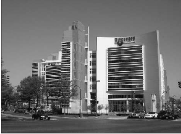
Photo 12.1. Discovery Communications Headquarters, Downtown Silver Spring, MD.
