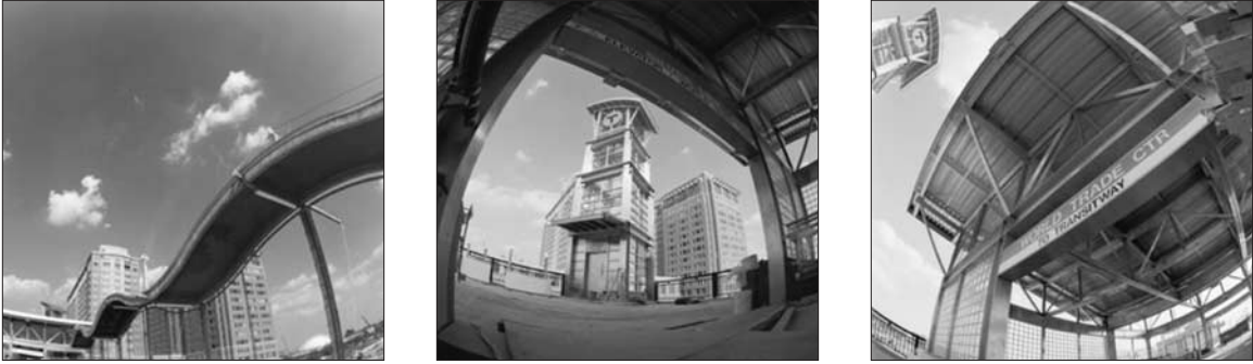
Photo 10.7. Views of the World Trade Center Silver Line Transit Stop.
