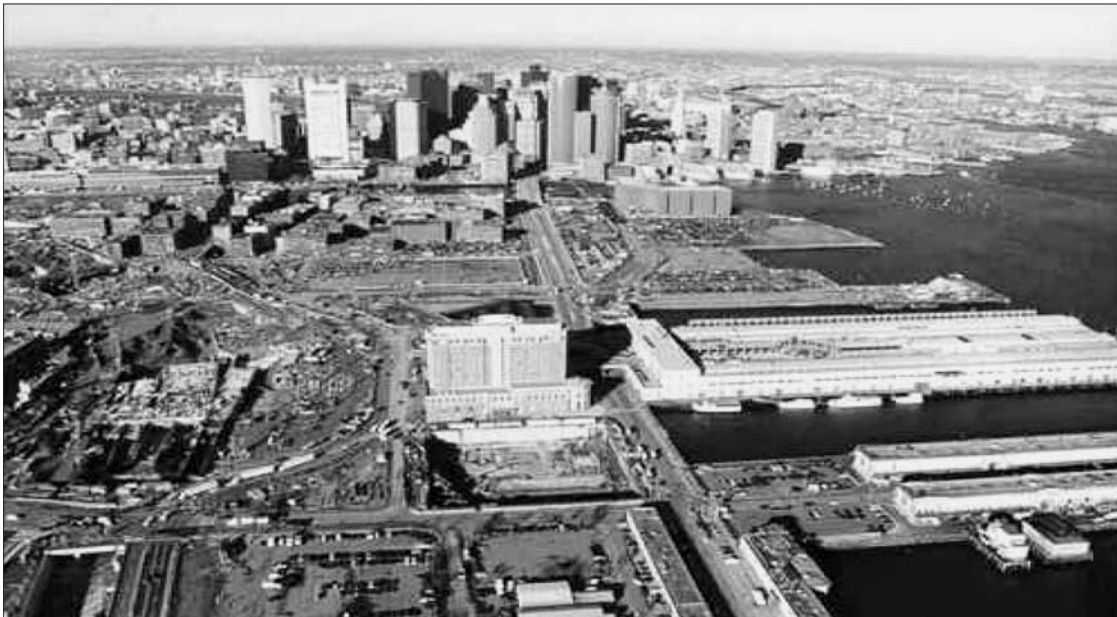
Photo 10.6. Aerial View of South Boston Waterfront. Opportunities for cities to start over again on such a large tract of land so close to the central core are rare indeed. Boston has ambitious plans to make the Seaport District the crown jewel of its TOD renaissance by making the District a high-density urban village and tourist attraction served by a multimodal transit system.
