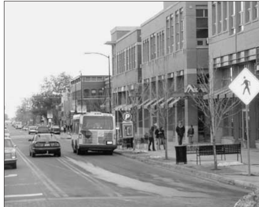
Photo 16.5. Mixed-Use Parking Structures in Downtown Boulder. City-owned parking structures in downtown Boulder are “wrapped” with ground-floor retail uses to promote active street frontages conducive to transit ridership.
