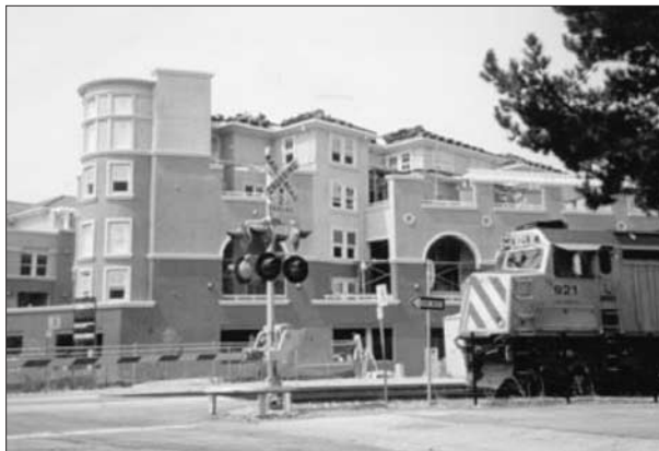
Photo 18.1. Franklin Street Project Taking Form at the Redwood City Caltrain Station.
