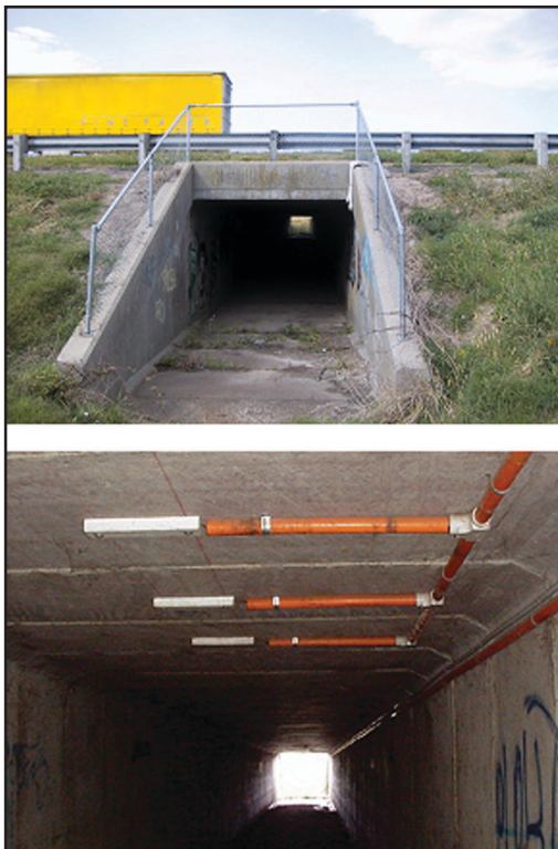
Figure 22. WIM sensors in situ.
