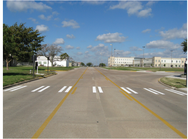
Figure 88. Example of bar pairs crosswalk markings
