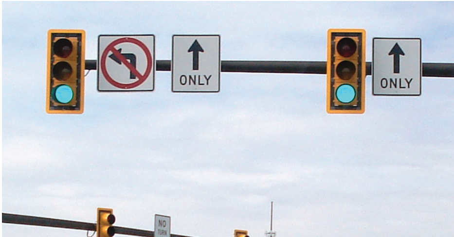
Figure 24. Yellow retroreflective backplates
