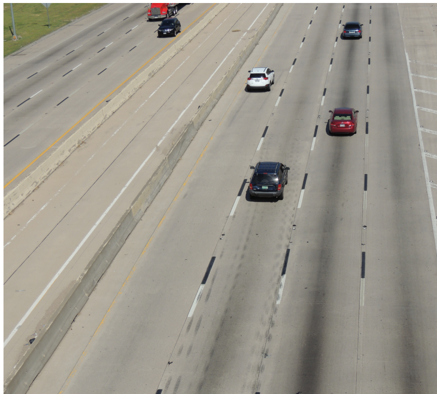
Figure 57. Contrast Markings on Light Colored Pavement
