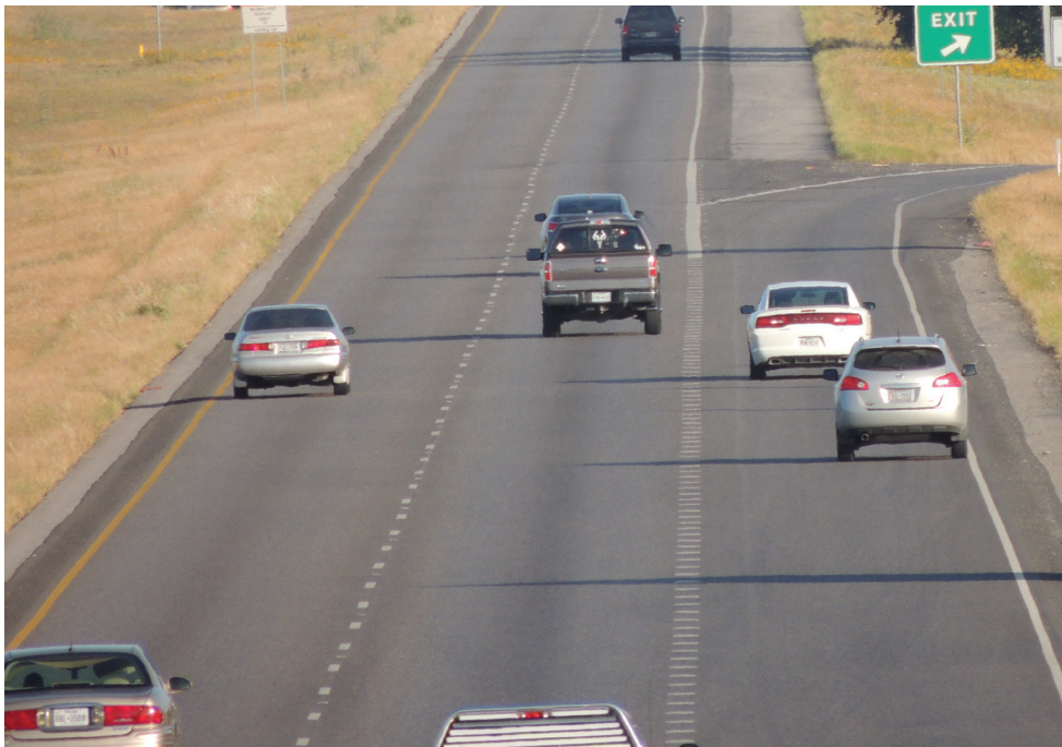
Figure 56. Dotted Lane Line Markings at Freeway Lane Drop
