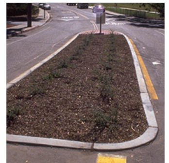
Figure 7. Vertical Curb (top), Sloping Curb (bottom)
