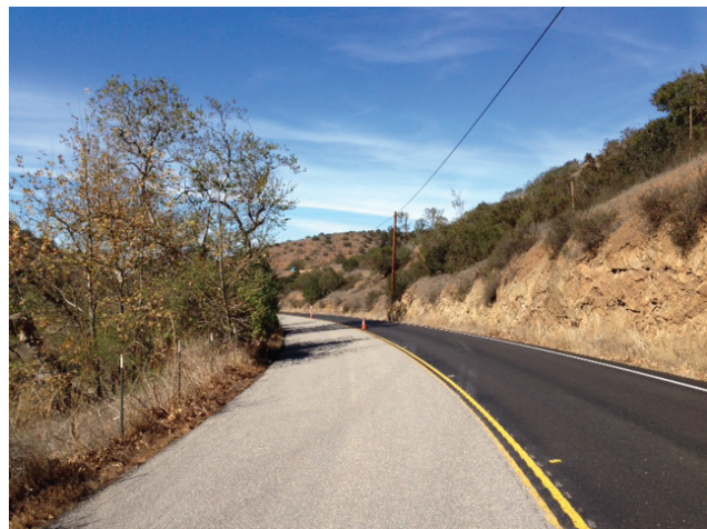
Figure 60. High Friction Surface Treatment on a Horizontal Curve
