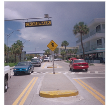
Figure 11. Raised median island with yellow marking on the vertical face and top surface
