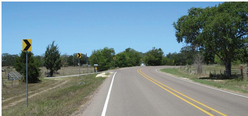
Figure 51. White edge lines, centerline RPMs, and chevrons on a horizontal curve
