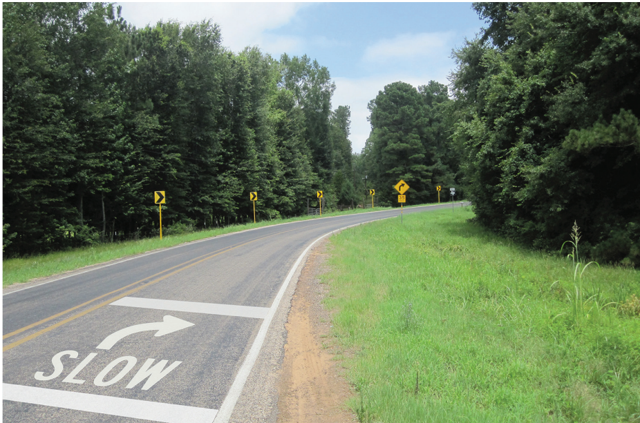
Figure 58. Curve Warning Markings ( MUTCD :5)
