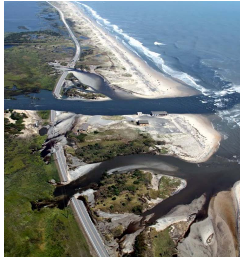
Three breaches in NC12 after Hurricane Irene. Credit: Tom MacKenzie, FWS
