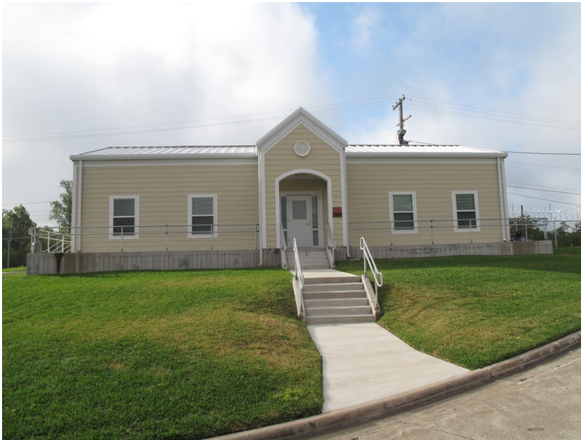
Troy Dent Fleet Operations Building Beaumont, Texas
