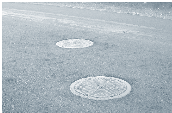
Figure 19. Handwork with WMA around manhole.
