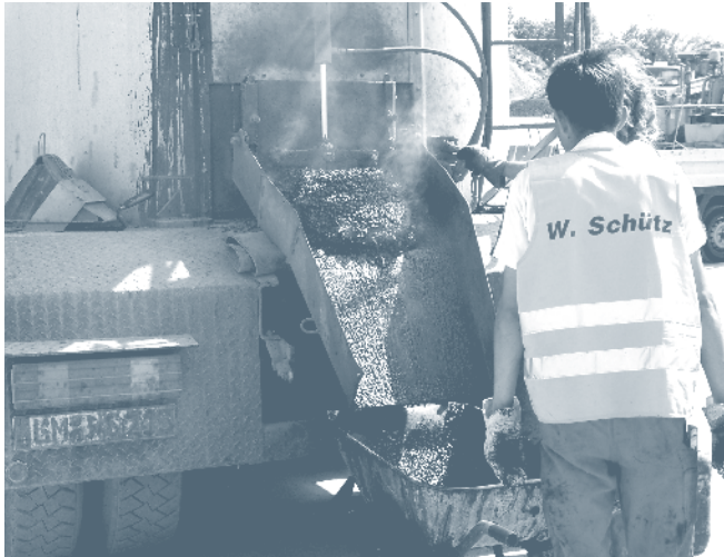
Figure 20. Unloading a mastic asphalt transport.
