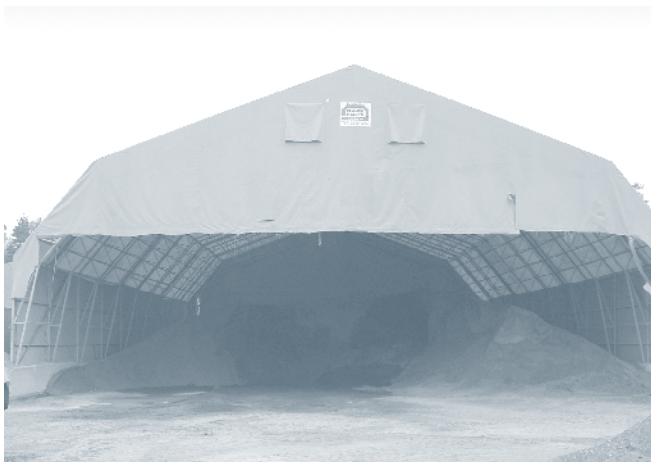
Figure 16. Kolo Veidekke's covered RAP storage.
