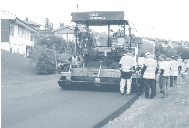
Figure 17. Heavy tamping-bar paver.
