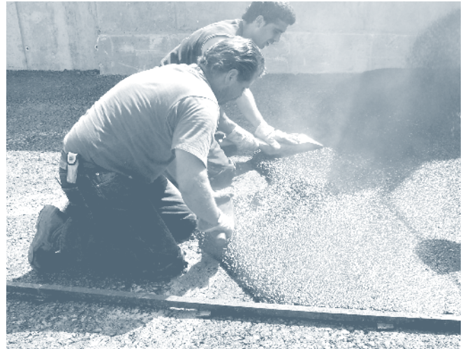
Figure 21. Placing mastic asphalt.
