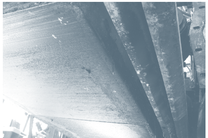
Figure 18. Close-up of tamping bars and vibratory screed.
