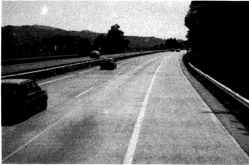
Figure 3.7 Photo of the AI recycled concrete pavement near Salzburg, Austria.
