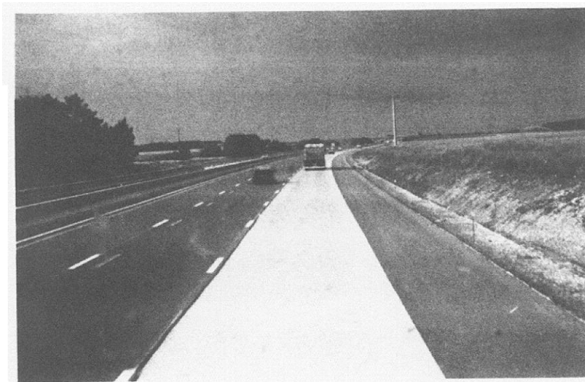
Figure 2.11 CRCP truck lane addition to original AC pavement in France.
