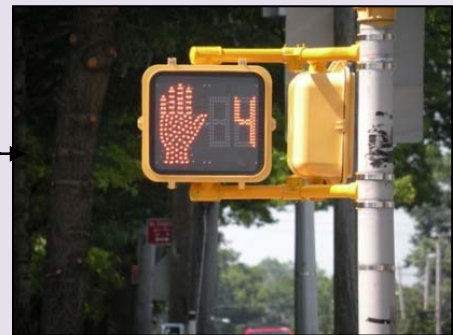
LPI, also known as a “pedestrian head start,” provides increased visibility and safety for pedestrians when drivers are turning, especially at right turns.
