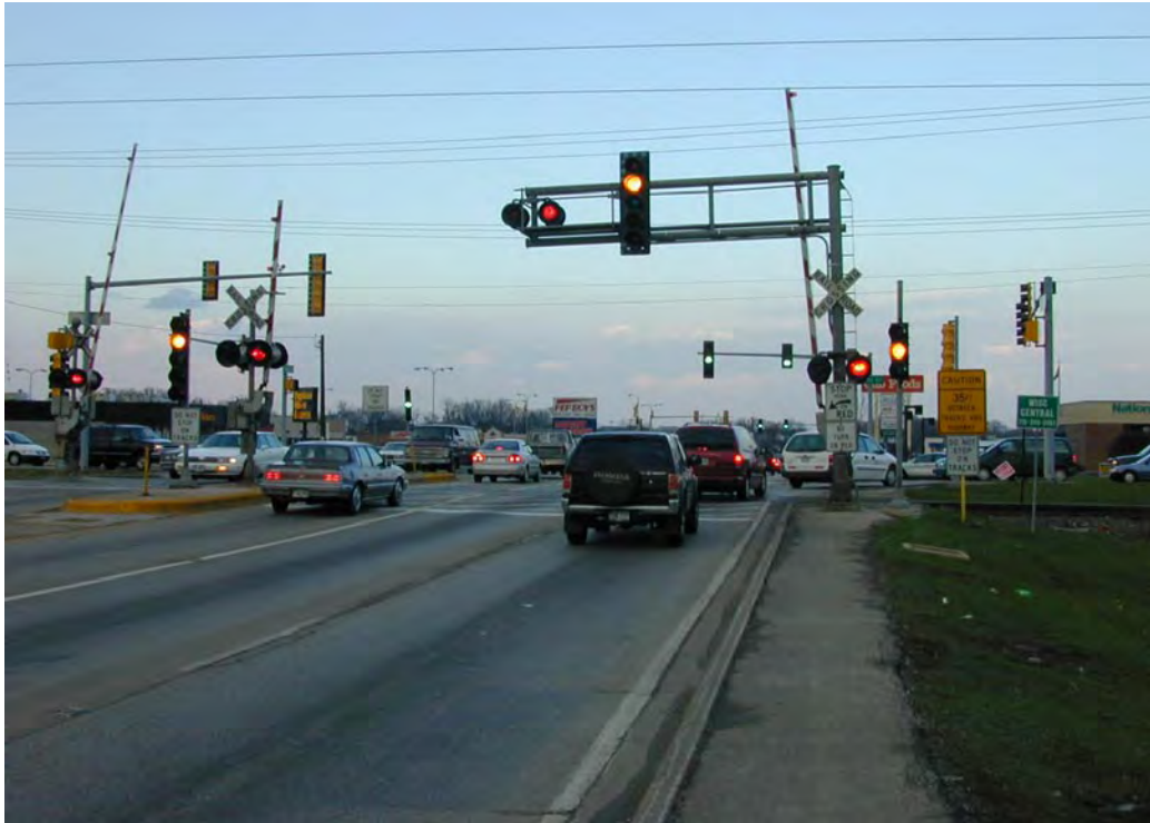
Figure 50. Pre-Signal Mounted on Railroad Cantilever, Rollins Road and State Route 83 at Wisconsin Central, Round Lake, Illinois
