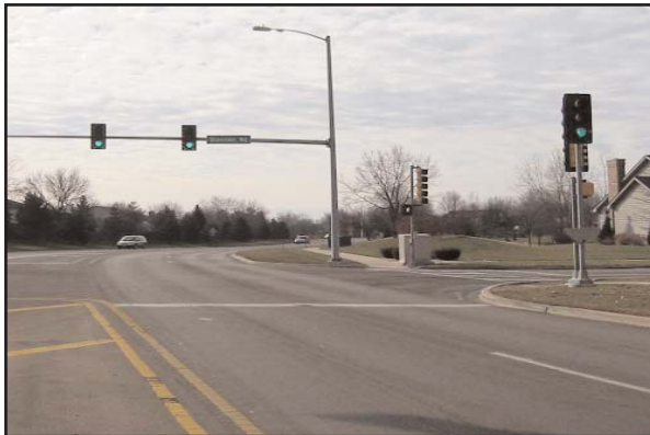
Figure 3-8. Two Overhead Signals for a One Lane Approach and Supplemental Pole Mounted Signal.
