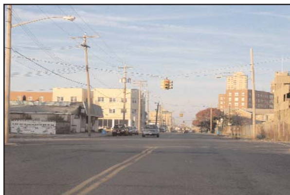
Figure 3–1. Intersection with One Signal Head (Non-compliant with the MUTCD).
