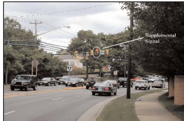
Figure 3-9. Approach View of Supplemental Signal on Near Side at Intersection.
