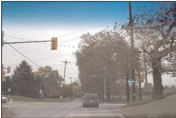
Figure 3–3. Posted-Mounted Signal no Longer Blocked by Vehicle.
