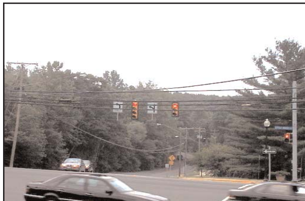
Figure 4-3. Example of Signal View Restricted by Utility Wires.
