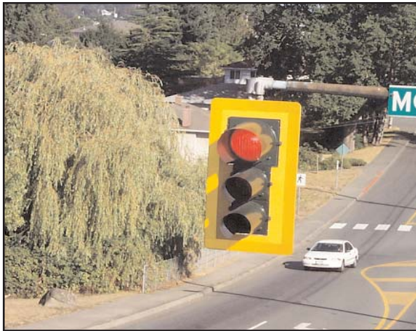
Figure 3–16. Signal with High Intensity Yellow Retroreflective Tape on the Backplate.
