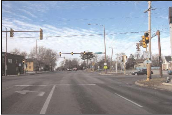
Figure 3-7. More Than One Primary Overhead Signal Per Lane, Plus Pole-Mounted Secondary (Left Side) and Tertiary Signal Heads (Right Side).
