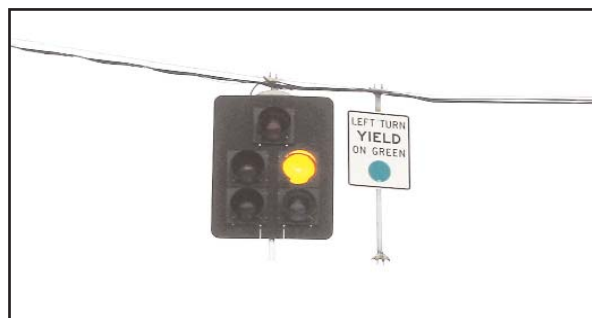
Figure 3–15. Traffic Signals with Backplates.
