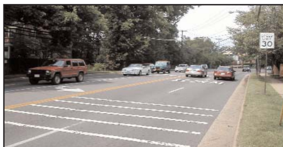
Figure 3–20. Rumble Strips and Pavement Markings Used to Alert Drivers of Signal Ahead.
