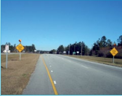
Figure 1: Through Vehicle Activated Warning Sign System warns through drivers of a vehicle on a cross street stop approach Photo Courtesy North Carolina DOT
