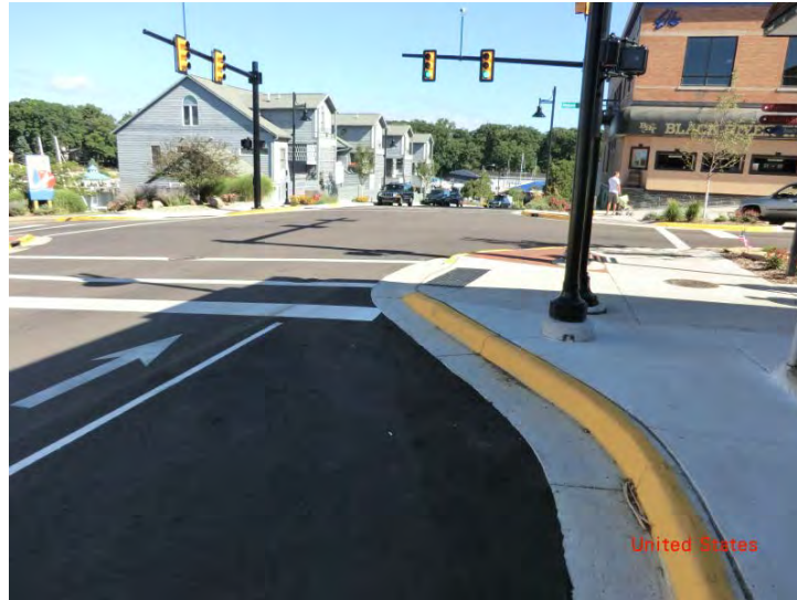
Exhibit 9-3. Intersection with curb extension in South Haven, Michigan. Photo credit: Jeff Shaw, Federal Highway Administration
