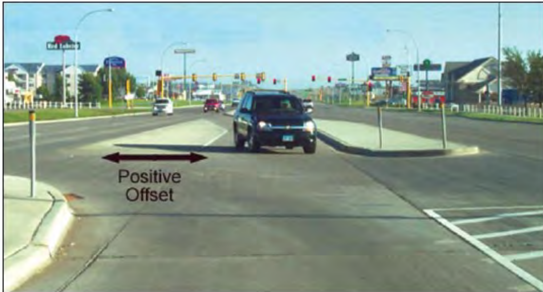
Exhibit 11-5. Example of positive offset left-turn lane.
