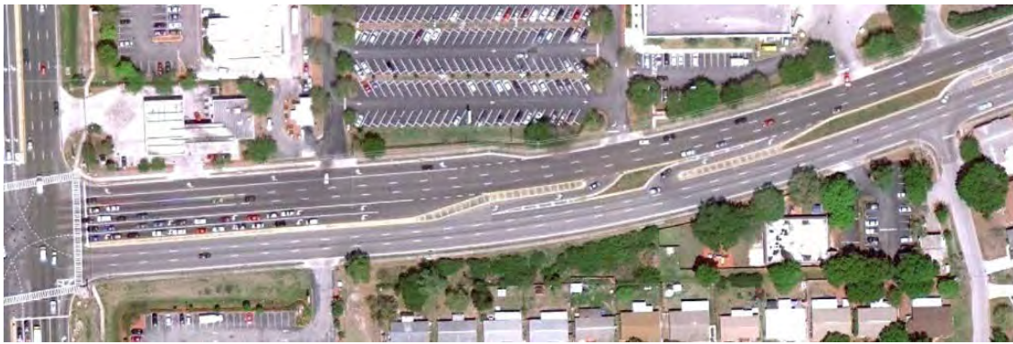
Exhibit 4-5. This raised median restricts left-turn egress movements from a driveway located between two intersections.
