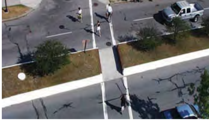
Exhibit 8-5. This refuge island enables two-stage pedestrian crossings.
