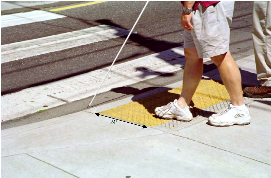
Exhibit 4-21. This crosswalk design incorporates the use of detectable warning surfaces into the curb ramps to facilitate navigation by a visually impaired pedestrian.
