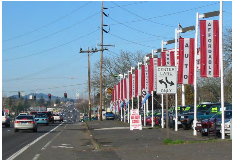
Exhibit 2-2. Example of sign clutter.
