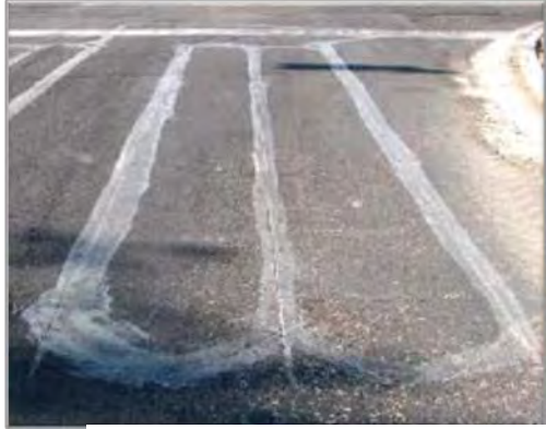
Exhibit 1-2. Vehicle detection by inductive loop (left) and video (right) (Source: Left: South Carolina DOT / Right: Jeff Shaw, FHWA)
