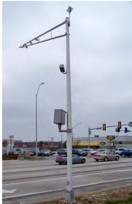
Exhibit 2-8. Enforcement cameras, as shown in the photo above, are used at signalized intersections to identify red light runners.
