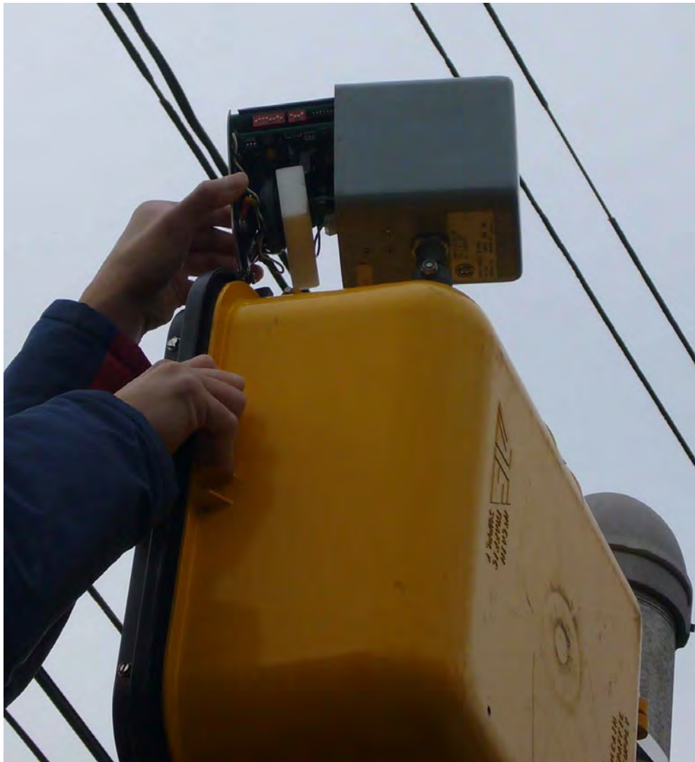
Figure 6-18. APS device with control board in pedhead (speaker opened for illustration).
