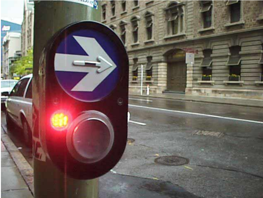
Figure 4-3. The tactile arrow above the pushbutton on this accessible pedestrian signal is superimposed on a larger visual arrow.
