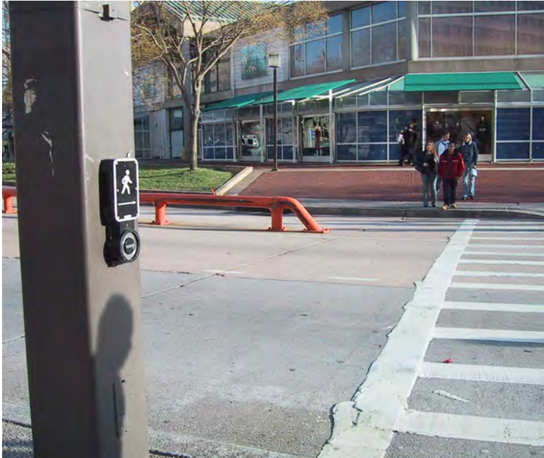
Figure 7-5. Well-located APS on a square pole.
