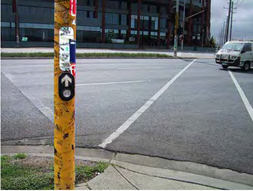
Figure 10-9. Installation of tactile arrows was not consistent and provided misleading information in some cases.
