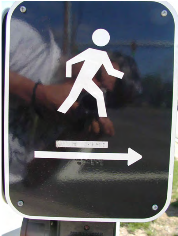
Figure 7-8. The faceplate at this location was mounted backwards, with the braille characters indented rather than raised and the small paper label, intended for translating the braille for the installers, is on the outside rather than the inside.
