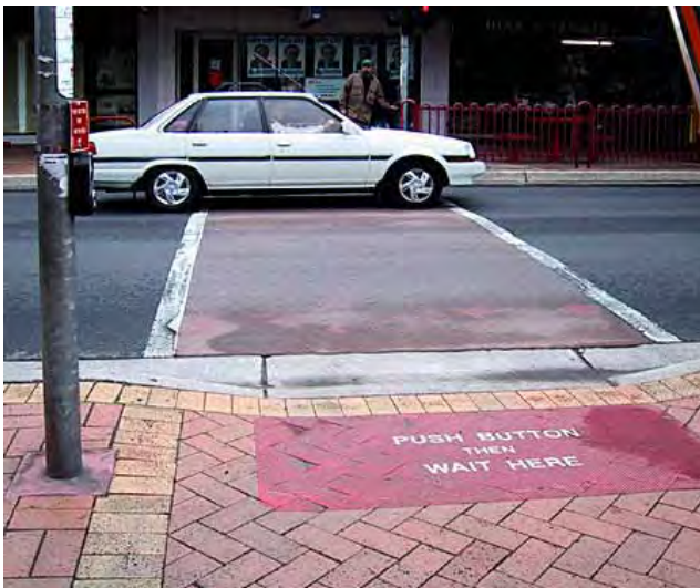
Figure 4-11. This midblock crossing has sensors in a specific area of the sidewalk. A red mat area is labeled “Push button then wait here.”
