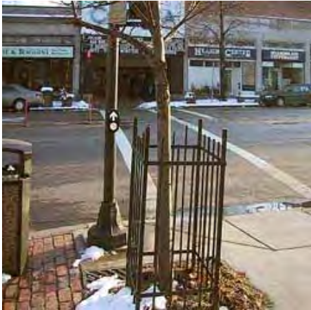
Figure 9-5. Panich APS at midblock crossing, Newton, MA. The APS should have been mounted on the side of pole closest to the crosswalk, with the arrow parallel to the crosswalk rather than pointing up.
