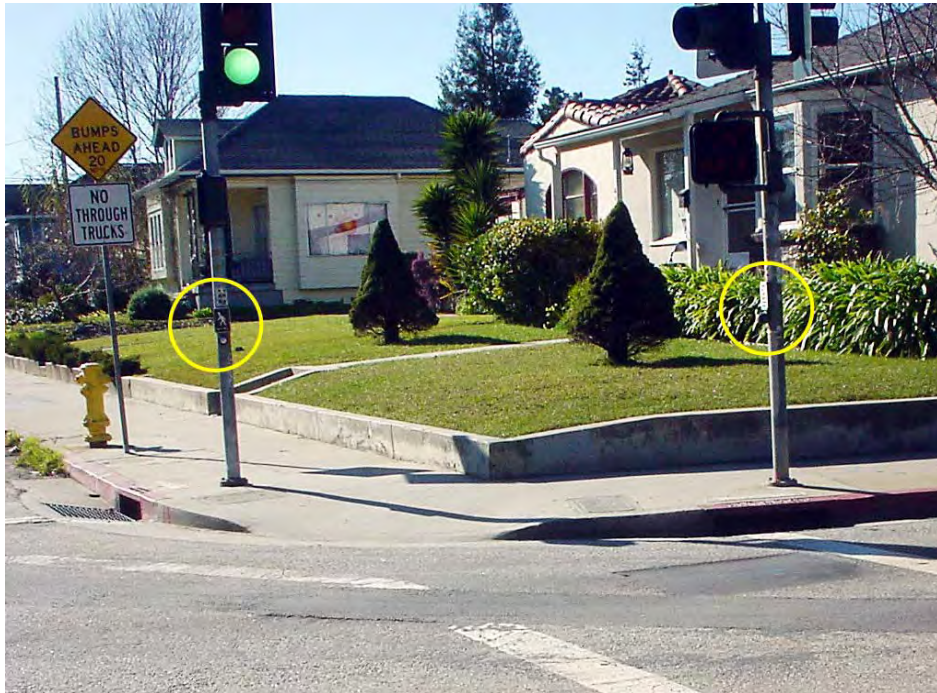
Figure 6-15. Well-located pedestrian signal poles provide APS audible indications from the optimal location, close to the pedestrian waiting area.
