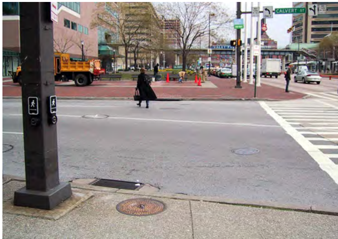
Figure 6-14. If pedestrians proceed directly to the curb from the pushbutton in this photo, they will be well outside the crosswalk area when beginning their crossing.
