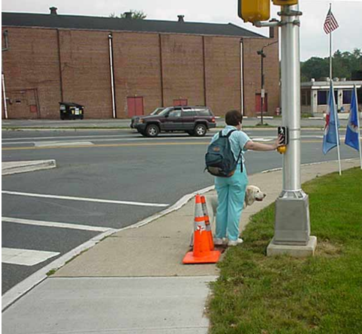
Figure 9-9. APS mounted on signal pole for crossing signaled right-turn lane. A pedestrian who is blind is waiting with her hand on the pushbutton for the vibrotactile “Walk” indication. After the “Walk” indication begins, she must turn and cross the sidewalk before beginning to cross the street.
