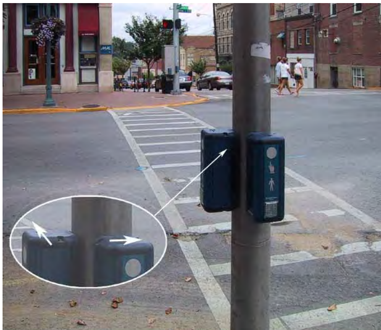
Figure 9-10. Mounting of two Prisma pushbutton units on a single pole. See arrows on insert detail for the orientation of the tactile arrow on the top of each unit. Both devices make the same sound during the “Walk” indication, which is acceptable in this installation since there is exclusive pedestrian phasing.
