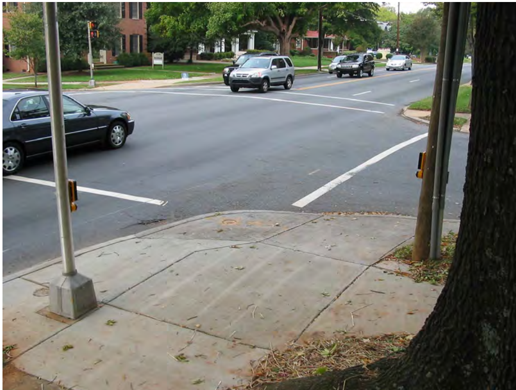
Figure 6-10. The APS should be located on the intersection side of the pole, as shown in this photo.
