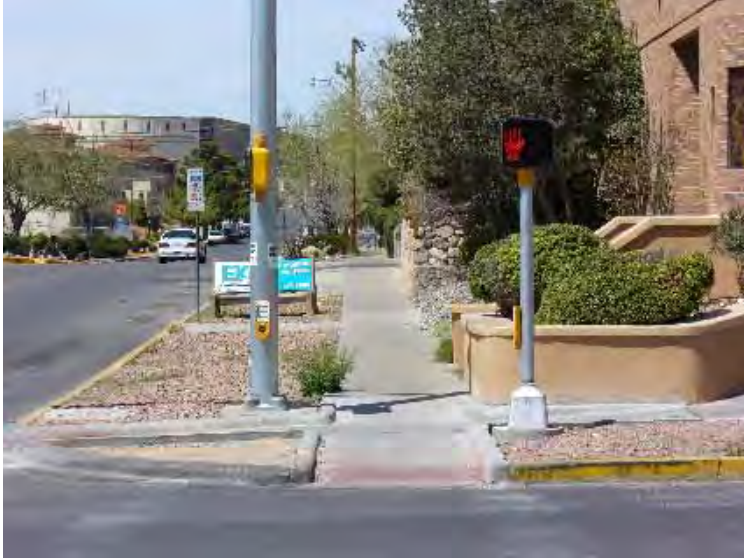
Figure 7-16. APS pushbuttons installed correctly.
