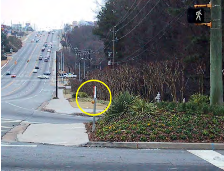
Figure 6-28. A stub pole is used to locate the pushbutton beside the sidewalk.
