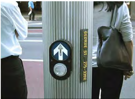
Figure 4-9. Example from Australia: a sign with raised print and braille characters is mounted vertically on a round pole to the right of an accessible pedestrian signal. The sign reads “GEORGE ST. 275-339R.”
