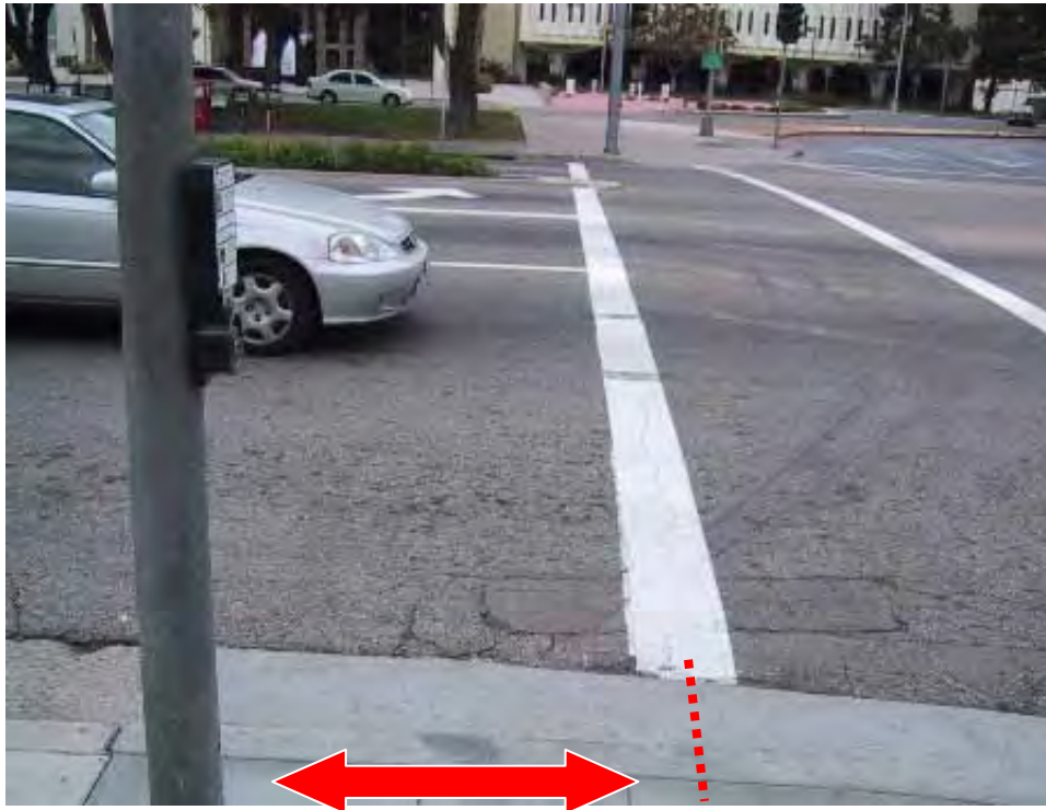
Figure 6-11. The MUTCD states that the APS should be within 5 ft of the crosswalk line extended.
