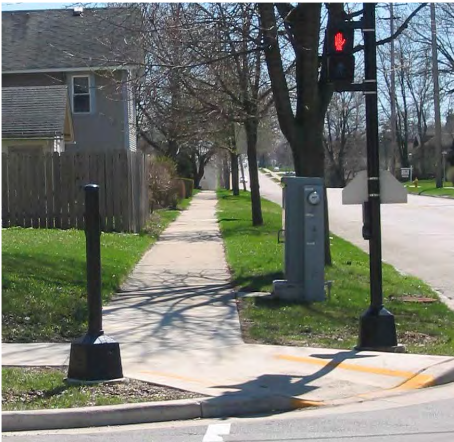
Figure 6-31. Stub pole example.
