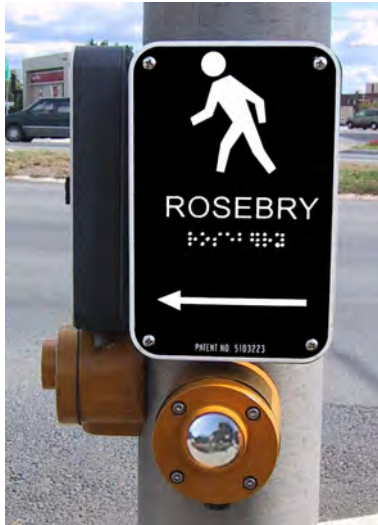
Figure 6-32. Braille label is below the raised print street name.
