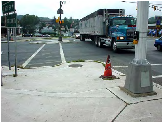
Figure 9-8. Installation of two pushbuttons on a single pole (only a single pushbutton is visible in the photo). Although the pushbutton is in line with the crosswalk, the pedestrian must travel more than 10 ft before reaching the street and the beginning of the crosswalk.
