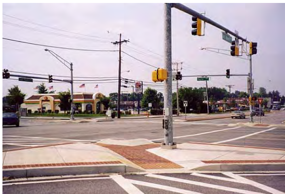
Figure 9-13. APS as seen from right-turn lane crossing.
