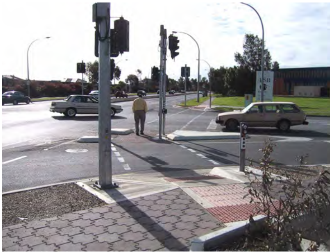
Figure 10-6. Signalized left-turn lane with APS mounted close to the crosswalk locations. Three APSs are on the splitter island, one for each crossing.
