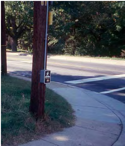
Figure 9-17. An early Polara installation in Charlotte.
