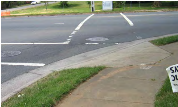
Figure D-3. Photo and sketch of an apex ramp configuration.
