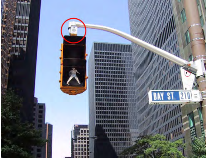
Figure 6-4. The mast arm is used in this installation in Toronto, Canada, to position the pedestrian signal head and speaker closer to the crosswalk.
