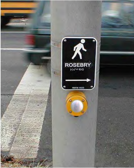
Figure 4-8. A braille street name is included on a sign above the pushbutton. The street name is also provided in high contrast large print (but not raised print) at this location.
