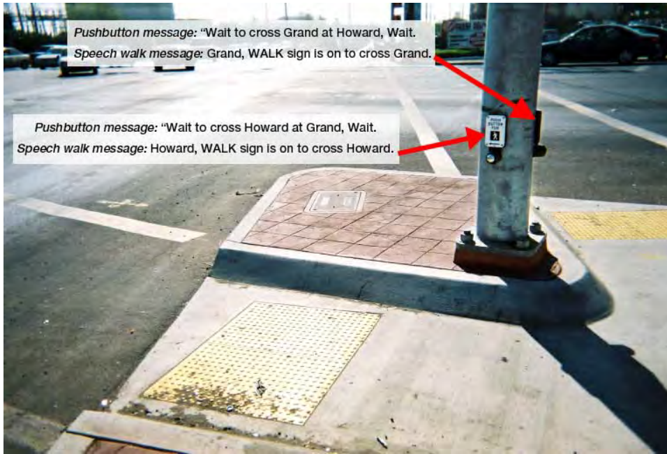
Figure 6-52. Example of pushbutton information messages and speech “Walk” messages for two APSs located on the same pole.
