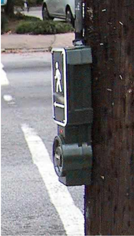
Figure 6-23. When the APS is mounted on a wooden pole, an additional mounting bracket is installed to allow the wires to run from the conduit into the top of the pushbutton-integrated device.
