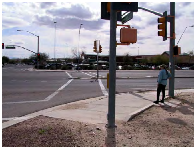
Figure D-7. This crosswalk is defined as skewed because it is timed for median crossing (two-stage), and a blind pedestrian might miss the median due to the bent crosswalk.
