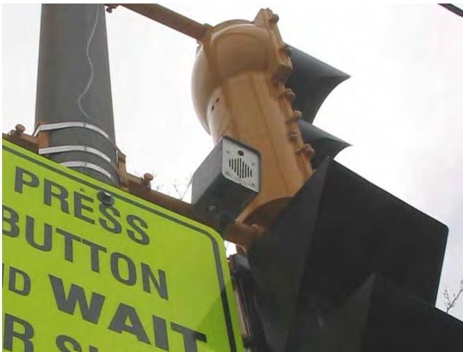
Figure 9-21. APS speaker mounted on signal head support arm.
