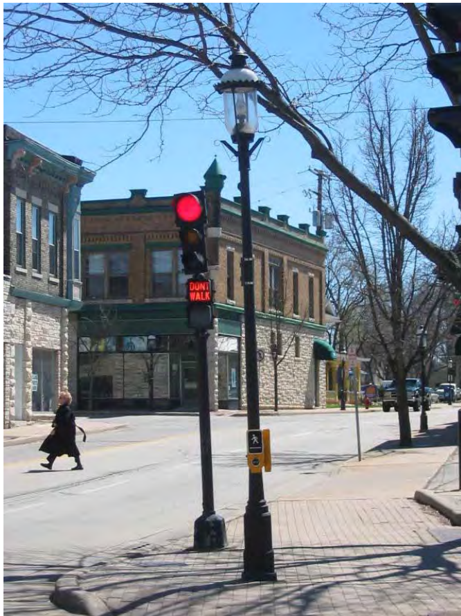
Figure 9-22. APS mounted on lamppost.
