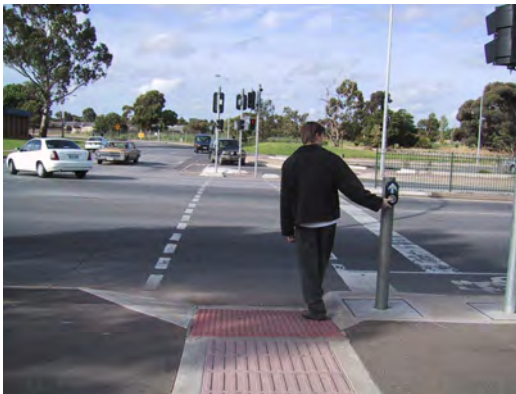
Figure 10-8. Typical APS location in relation to the crosswalk and sidewalk. Australian curb ramp standards allow a steeper slope than allowed by U.S. standards.
