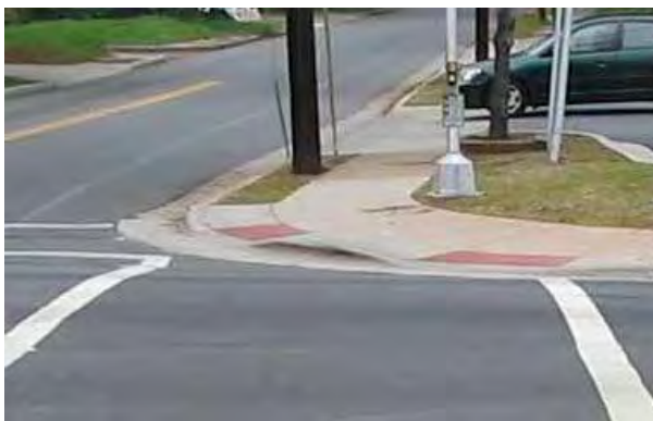
Figure D-4. Photo and sketch of a perpendicular ramp configuration.
