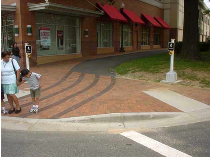
Figure 9-1. Pushbutton-integrated APS located on a stub pole beside the level landing of the curb ramp.
