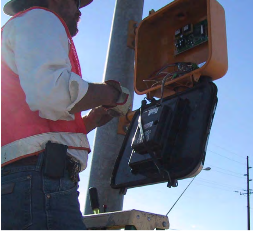
Figure 7-2. Technician installing APS control board in pedhead.
