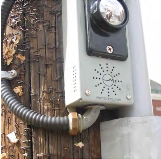
Figure 9-20. APS pushbutton mounted on wooden pole, showing conduit installed into the bottom of the pushbutton device.
