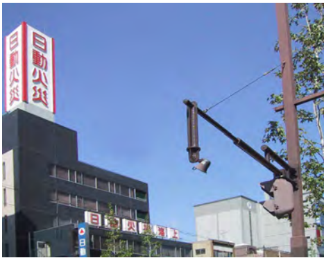
Figure 10-3. Pedhead with APS speaker is mounted on a mast arm overhanging the crosswalk below.
