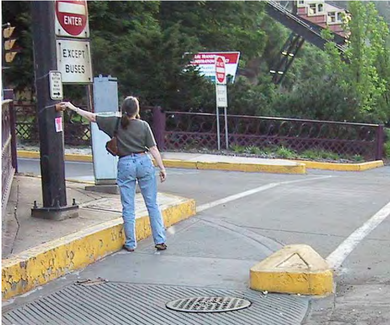
Figure 7-3. This pushbutton may be 42 in. from the bottom of the pole, but it is almost 60 in. above the landing, making it inaccessible to a wheelchair user and not likely to be located by a person who is blind.
