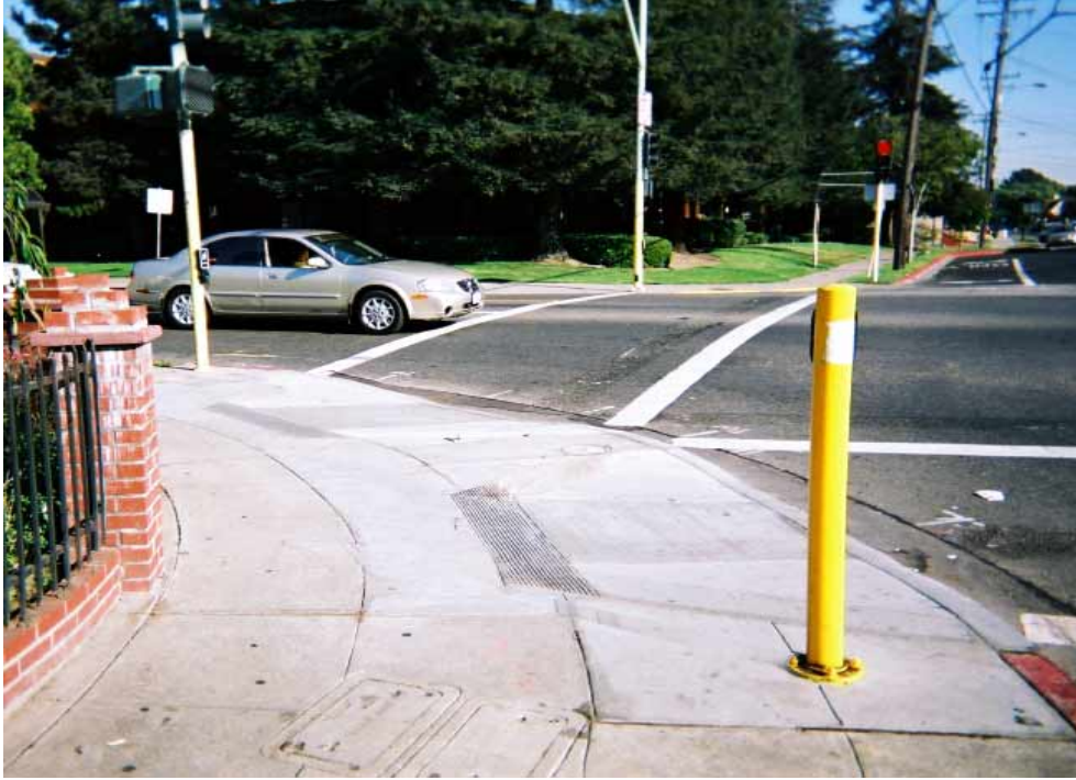
Figure 6-16. APSs are positioned appropriately at this intersection by the addition of a stub pole for one crosswalk. The stub pole holding the APS for the crosswalk at right is simply bolted to the sidewalk. The other APS is mounted on the pole that supports the pedhead.
