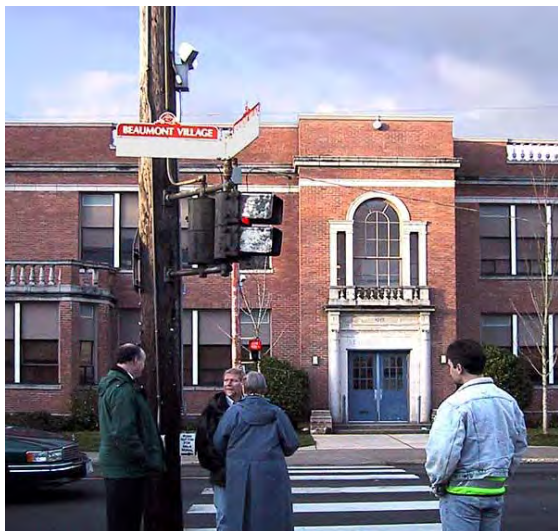
Figure 9-3. An APS mounted over 12 ft high on the pole broadcast speech messages at this location in Portland. City engineers expressed concerns about intelligibility of the message.
