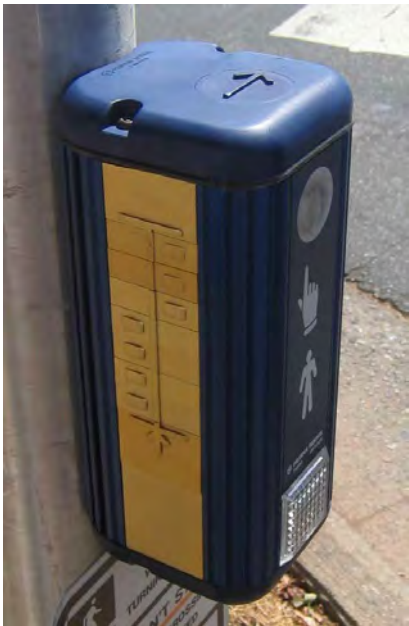
Figure 4-4. The tactile arrow is located on top of this APS housing (note the lack of required color contrast between the arrow and housing).
