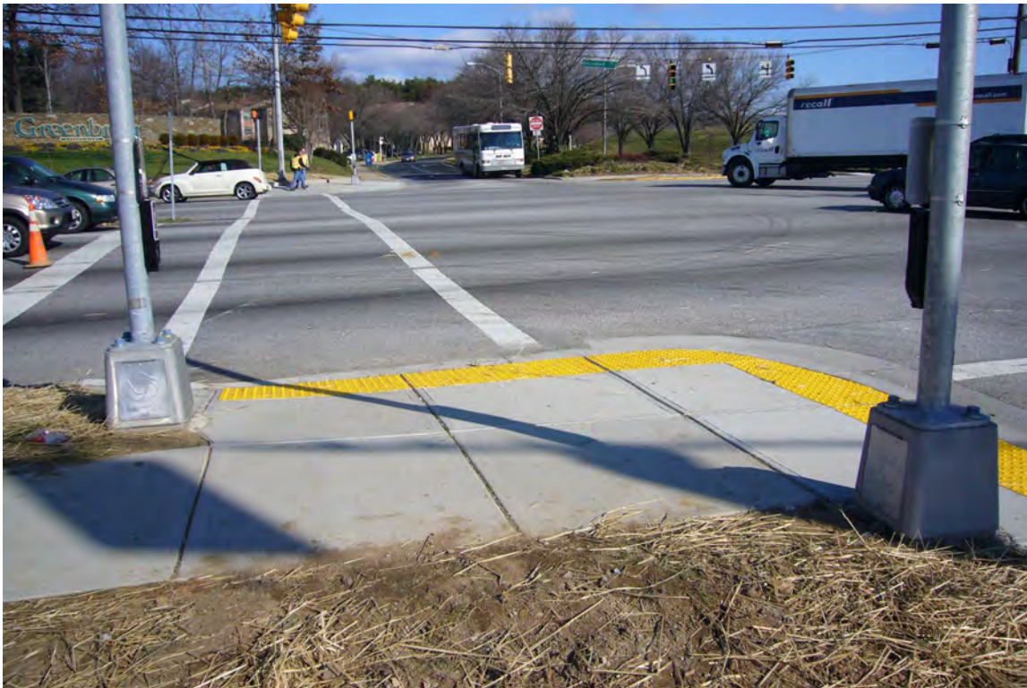
Figure 6-7. APS installation in new construction.
