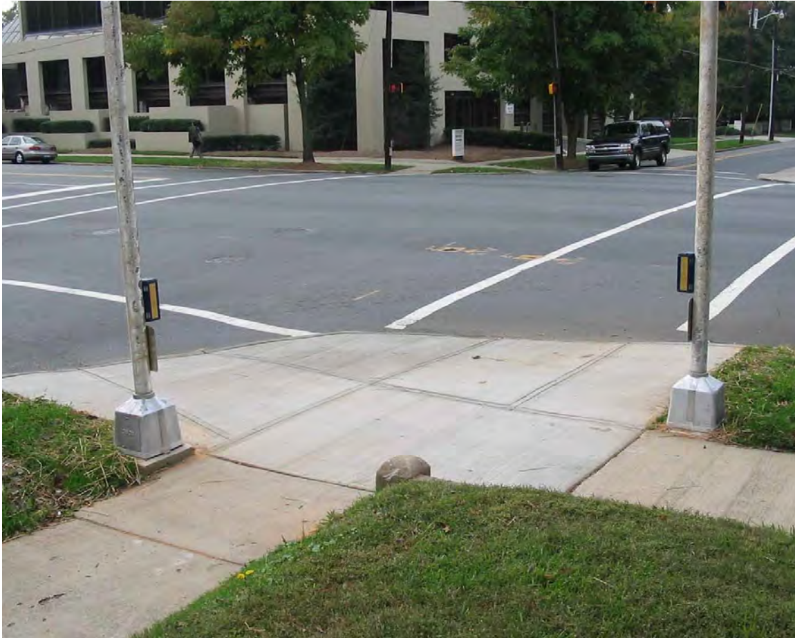
Figure 6-13. APSs installed in this reconstruction location are in accordance with the Draft PROWAG in that they are beside a level landing and separated from each other by at least 3 m. Both APS devices are located on the intersection side of their poles.
