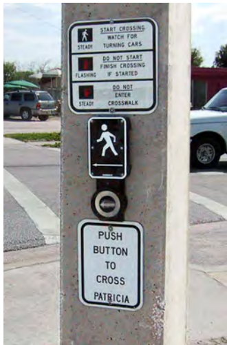
Figure 7-6. A mounting bracket or shim is needed on this square pole to properly orient the arrow . Without it, the arrow points to the center of the intersection.
