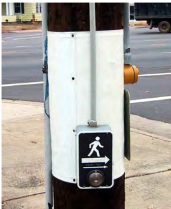
Figure 6-27. Coated canvas shield used in Charlotte, NC.
