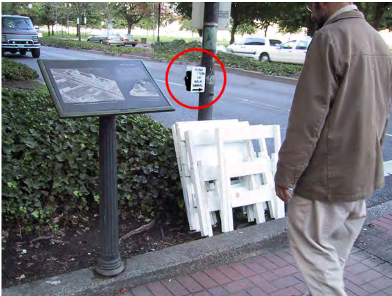
Figure 7-4. Not only is the pushbutton in the bushes and out of reach range from the sidewalk, but construction barriers have been stored against the pole, preventing all pedestrians from reaching the pushbuttons.
