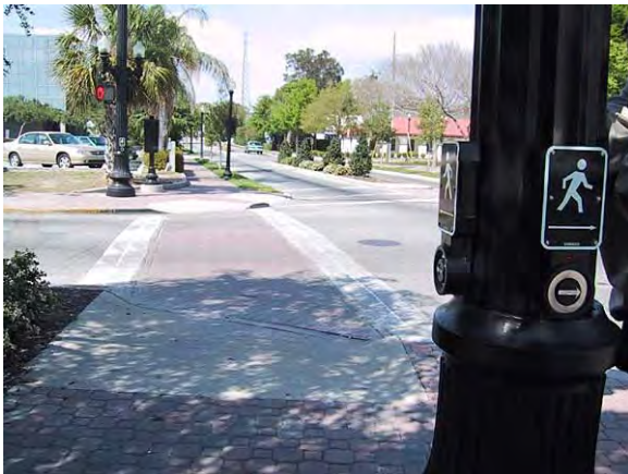
Figure 9-11. Two pushbuttons are located on fluted pole at this location with exclusive pedestrian phasing. Tactile arrow of each device points in the direction of travel on the crosswalk.
