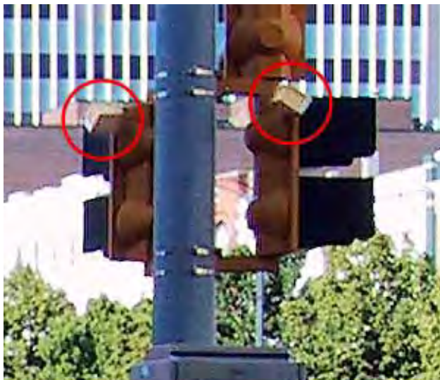
Figure 6-17. Two pedhead-mounted speakers, aimed at right angles to each other, are separated by the width of the pedheads and the mounting pole. More distance is preferred and careful aiming and volume control is important.
