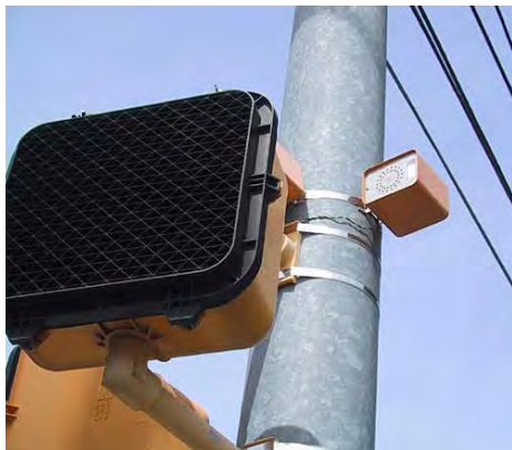
Figure 9-19. Pedhead-mounted speaker mounted on the pole as typically installed in Atlanta.
