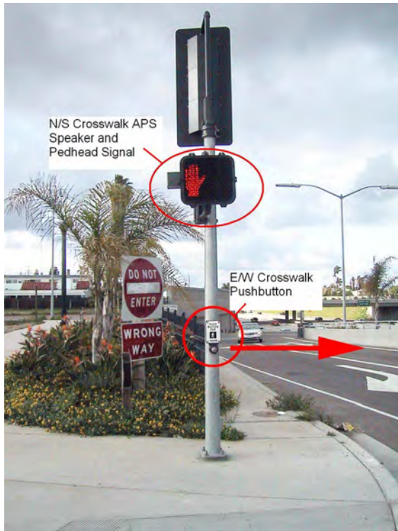
Figure 6-44. The pedhead and APS speaker for the north-south crosswalk is located over the pushbutton for the east-west crosswalk.
