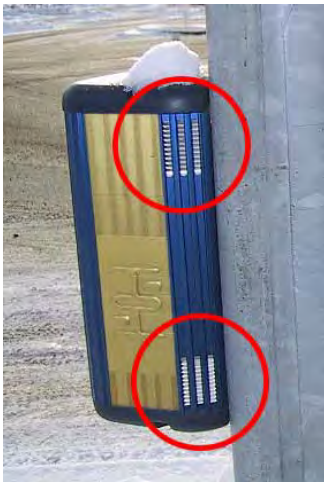
Figure 6-33. Speaker grille on side of APS.
