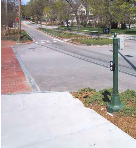
Figure 9-7. Panich APS on stub pole in Newton, MA. Arrow oriented parallel to crosswalk.
