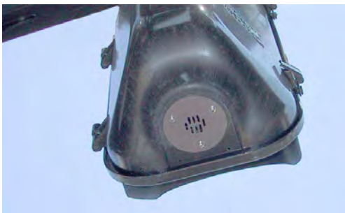
Figure 10-4. Japanese pedhead with APS speaker pointing straight down toward the pedestrian below.
