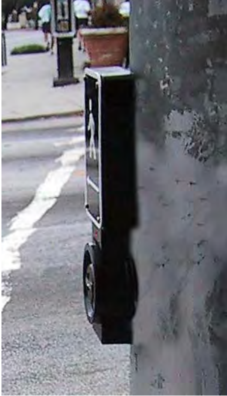
Figure 6-24. Typical installation without extra mounting plate, with wire running from inside the metal pole into the back of the device.
