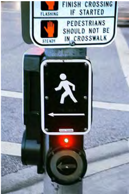
Figure 4-6. A red actuation indicator light is illuminated directly above the pushbutton.
