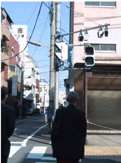
Figure 10-5. The PICS-A system is shown with four infrared transmitters mounted on a horizontal mast arm.
