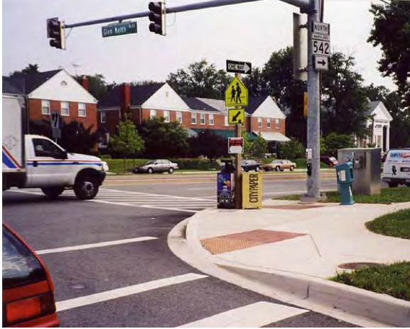
Figure 9-16. APS installed on signal pole beside crosswalk waiting location.
