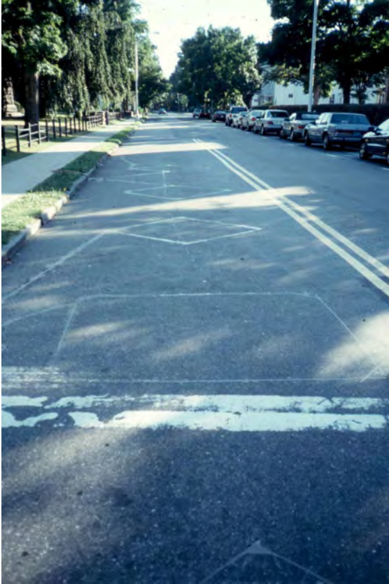
Figure 3-1. Vehicle detector loops in pavement.
