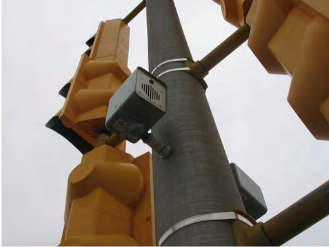
Figure 6-21. APS speaker mounted directly to the metal pole provides more support during high wind.
