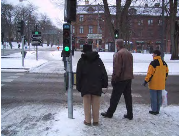
Figure 10-10. This intersection in Göteborg, Sweden, has a bike lane (seen on left side of photo) with its own signal head, and an APS is mounted on the same pole.
