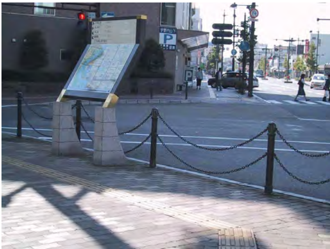
Figure 10-2. At this intersection, a chain fence is used where crossing is prohibited, and bar tiles indicate a travel route.
