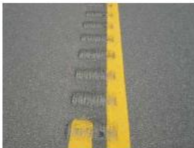
Figure 1a. Milled Rumble Strip/Stripe
