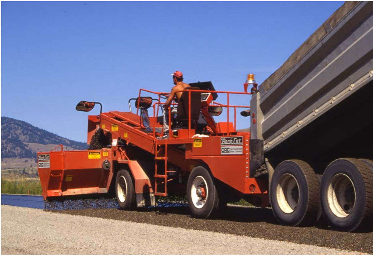
Exhibit 4-12 Chip Seal Aggregate Placement
