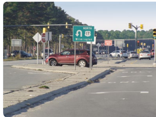
Vehicle Turning at an RCUT Intersection Along US 17 in NC Source: RCUT Video FHWA-SA-14-020
