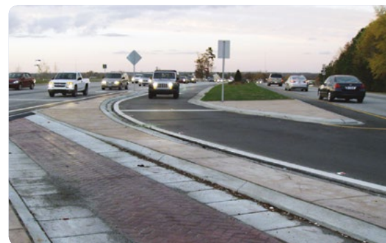
Vehicle Turning at an RCUT Intersection Along the NC 55 Bypass Source: RCUT Case Study Video FHWA-SA-14-063
