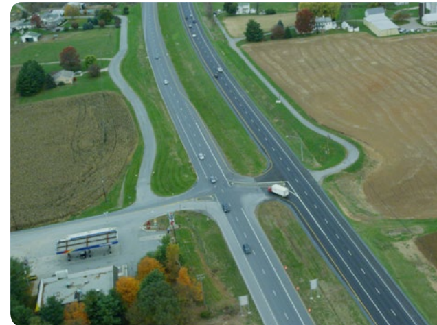
Frederick County, MD RCUT Intersection Source: RCUT Video FHWA-SA-14-020
