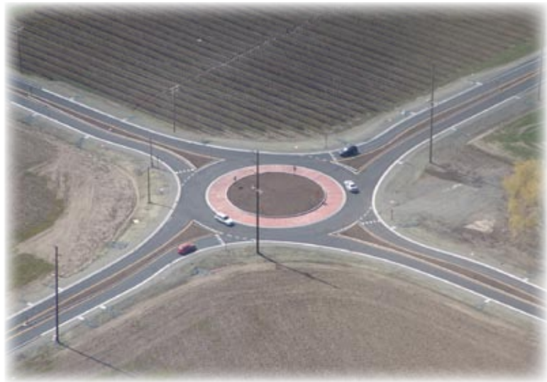
Figure 17: Use of Longer Splitter Islands in a Rural Environment (Skagit County, Washington)
