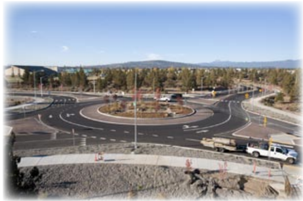
Figure 24: Example Markings for Multilane Roundabout (Bend, Oregon)
