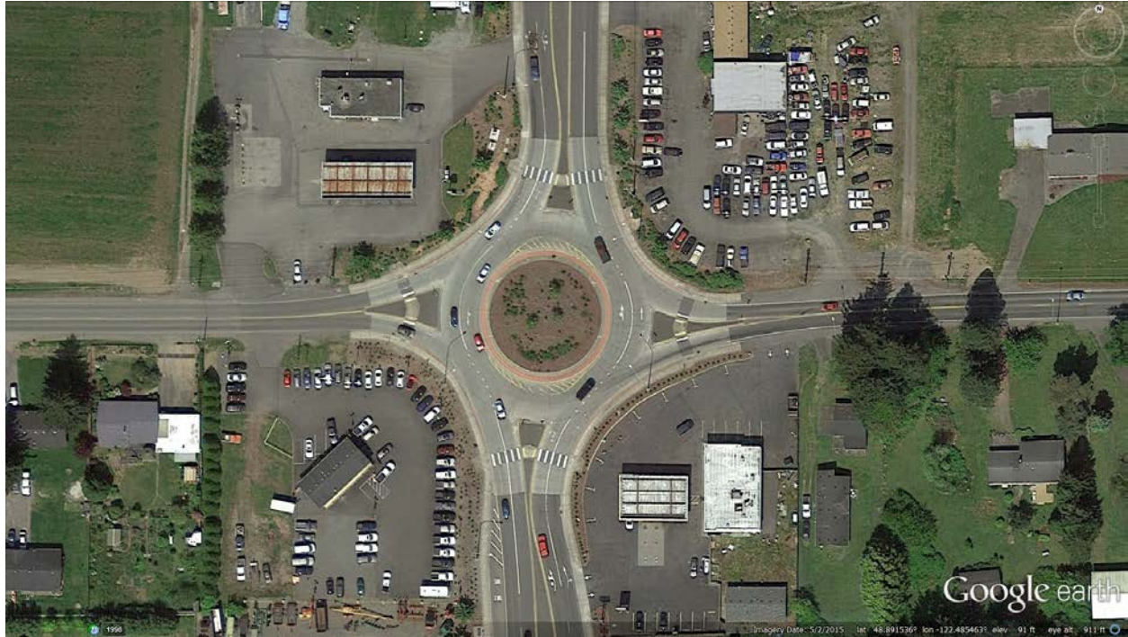
Figure 38. Photo. SR 539/Pole Rd., Lynden (Whatcom County), WA (Source: Google Earth 2015)
