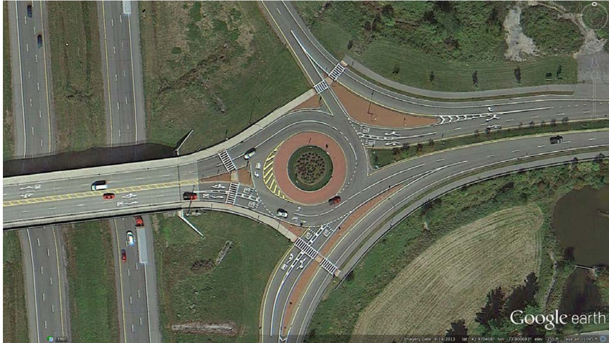
Figure 31. Photo. SR 67/I-87 NB Ramps, Malta, NY (Source: Google Earth 2013)
