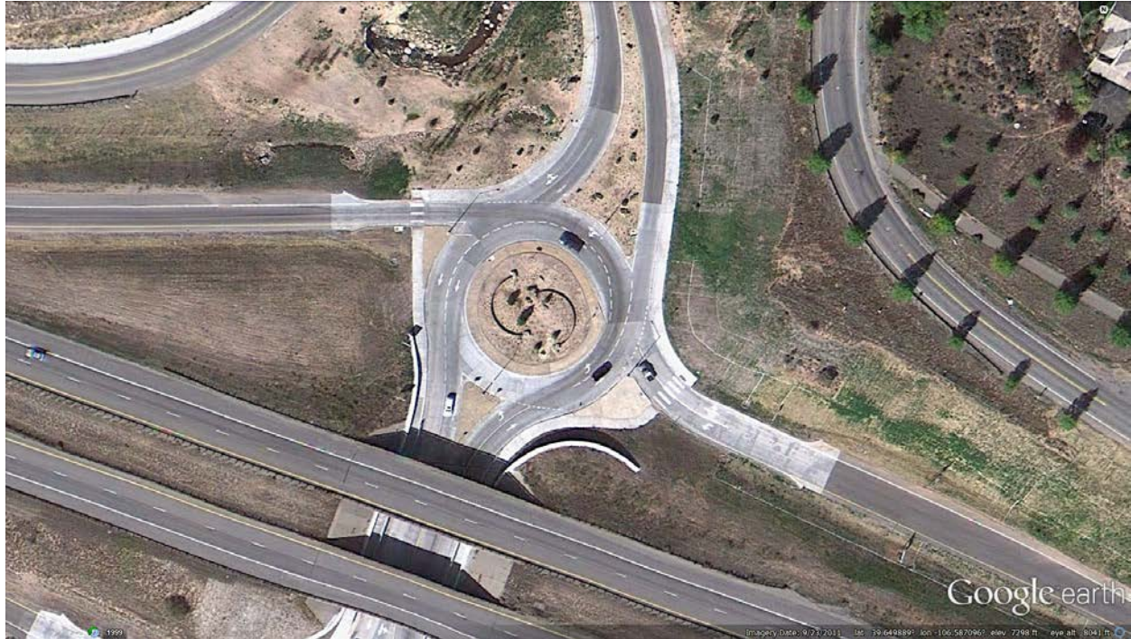
Figure 23. Photo. Edwards Access Rd./Beard Creek Rd./I-70 WB Ramps, Edwards, CO (Source: Google Earth 2011)
