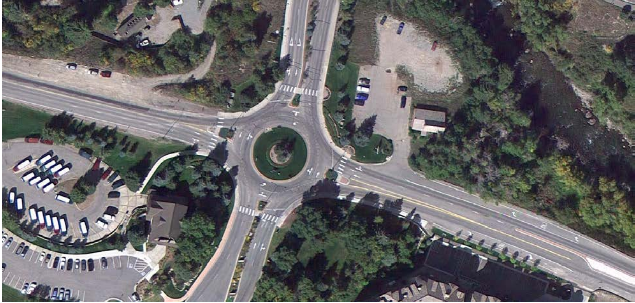
Figure 22. Photo. Avon Rd./US 6, Avon, CO (Source: Google Maps 2015)
