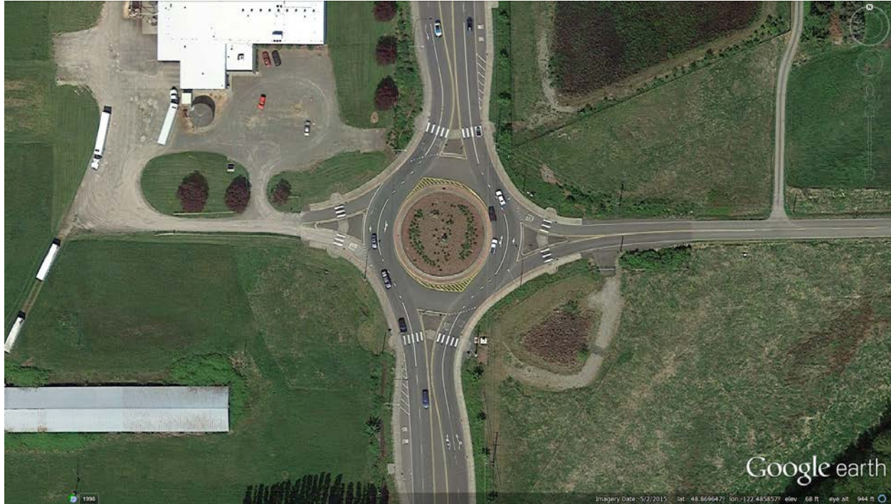
Figure 39. Photo. SR 539/Ten Mile Rd., Lynden (Whatcom County), WA (Source: Google Earth 2015)
