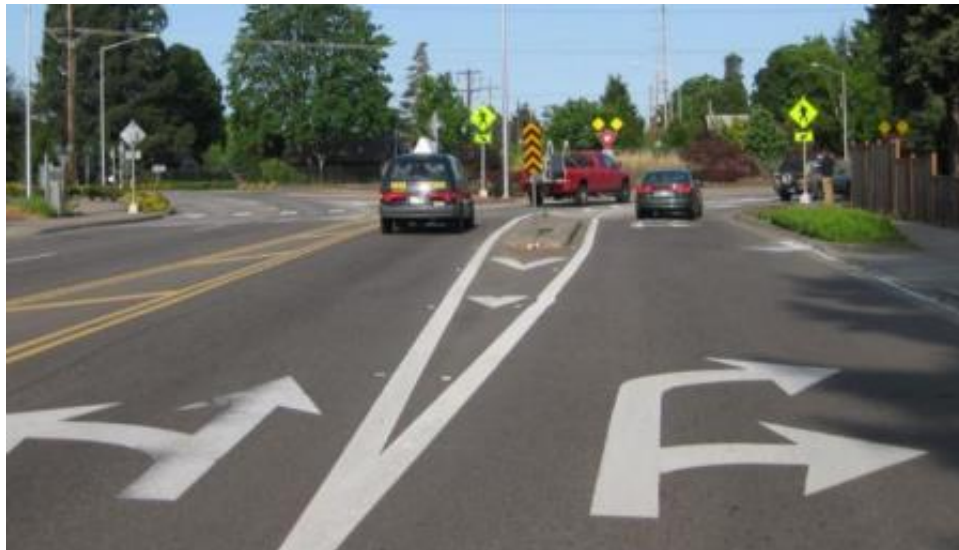
Figure 23. Photo. Hayden Bridge Rd. east leg two-lane entry, two-lane exit, Springfield, OR.
