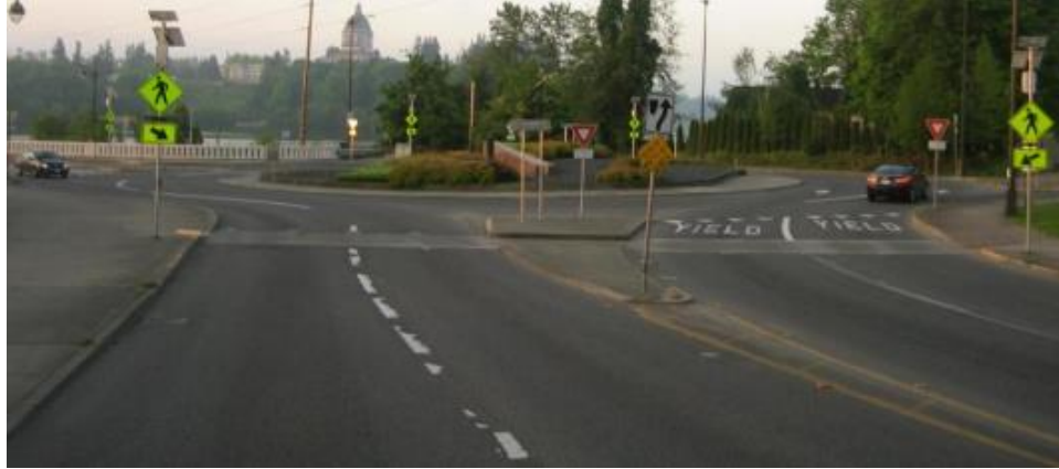
Figure 17. Photo. Olympic St. W, north leg two-lane Entry, two-lane exit, Olympia WA.
