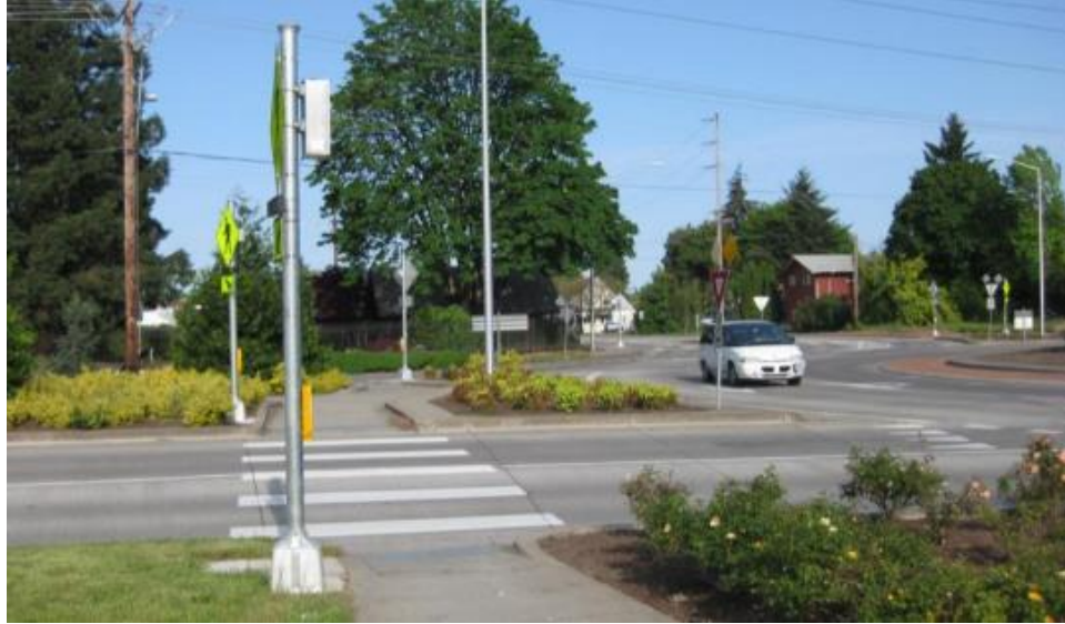
Figure 22. Photo. Pioneer Pkwy. south leg two-lane entry, two-lane exit, Springfield, OR.
