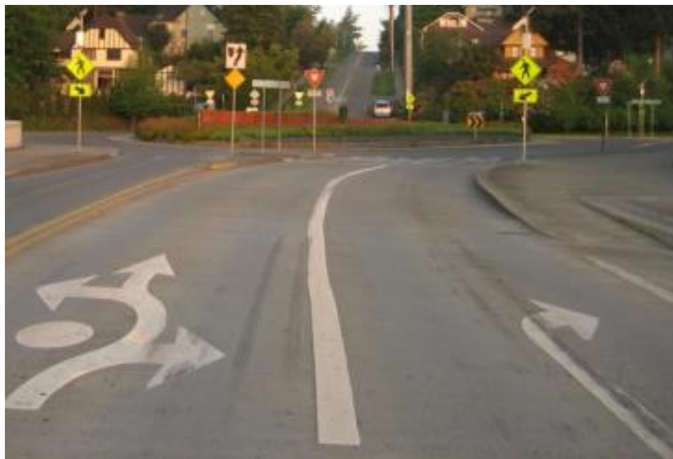
Figure 16. Photo. 4th Ave. W, east leg two-lane entry, one-lane exit, Olympia WA.
