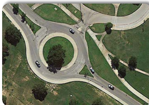
Figure 2: Roundabout at Auditorium Shores, Austin, TX Source: Google Earth Pro
