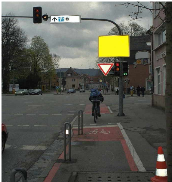
Fig 34: Design of the traffic flow system and the traffic light staggering system in favour of cyclists
