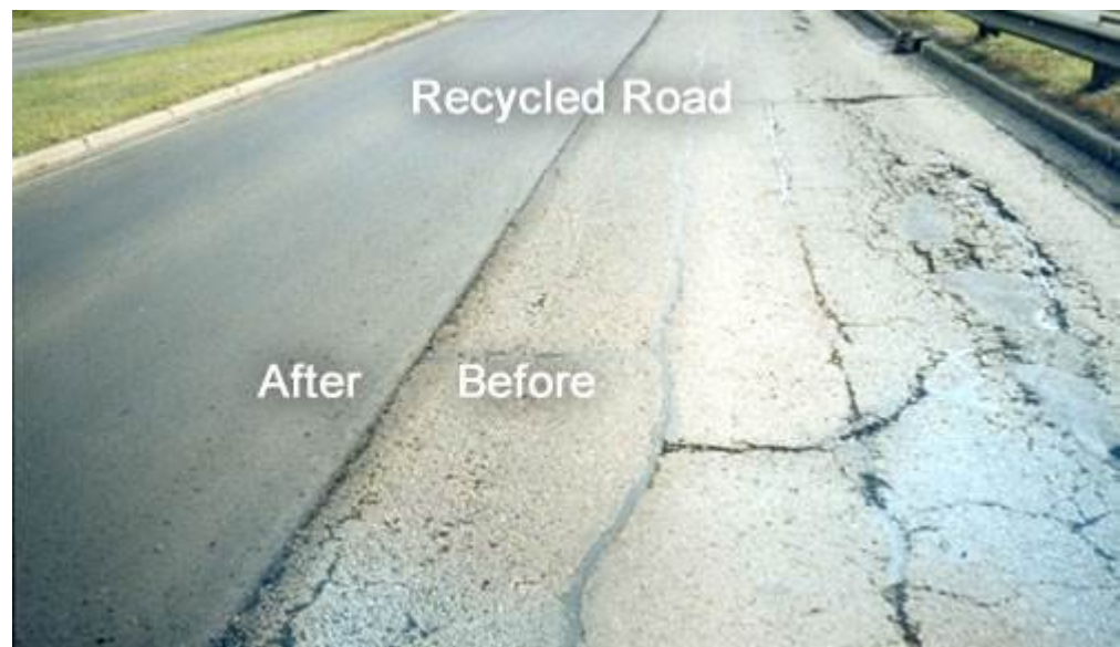
The impact of an asphalt recycling project on a road
